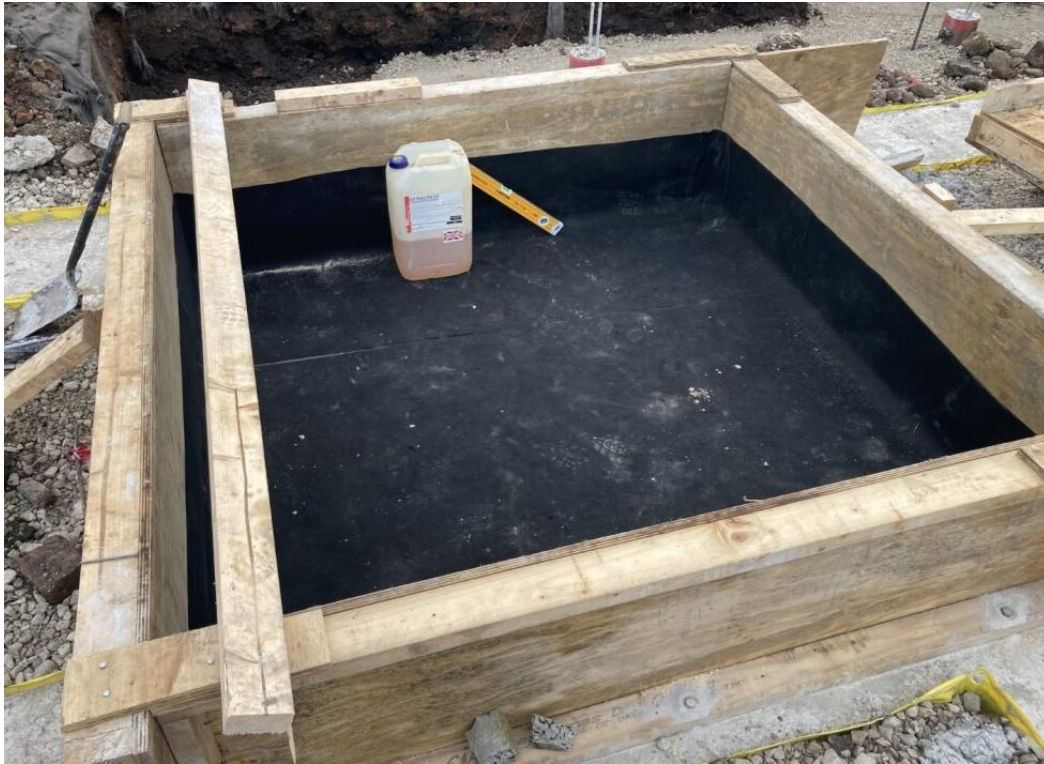
PLATE 4 INSTALLATION OF VAPOR GAS MEMBRANE
