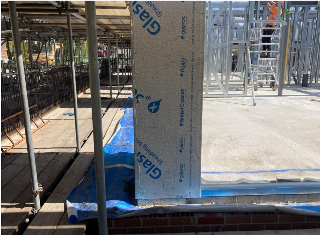
PLATE 5 BUILD PHASE WITH OVERHANG OF GAS MEMBRANE
