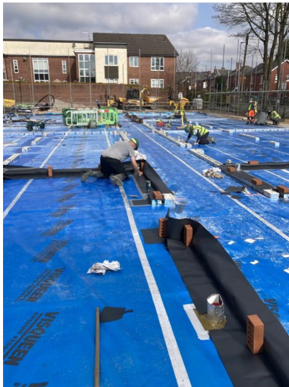
PLATE 4 INSTALLATION OF VAPOR GAS MEMBRANE
