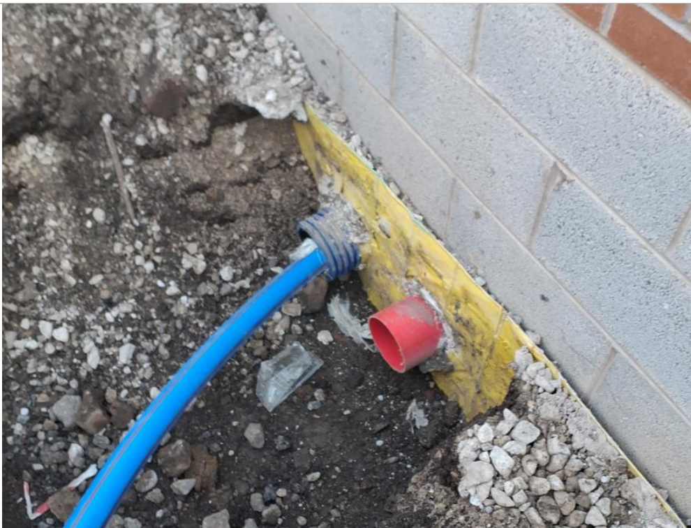
FIGURE 4.2 INSTALLED BARRIER (TYPE A) PIPEWORK
