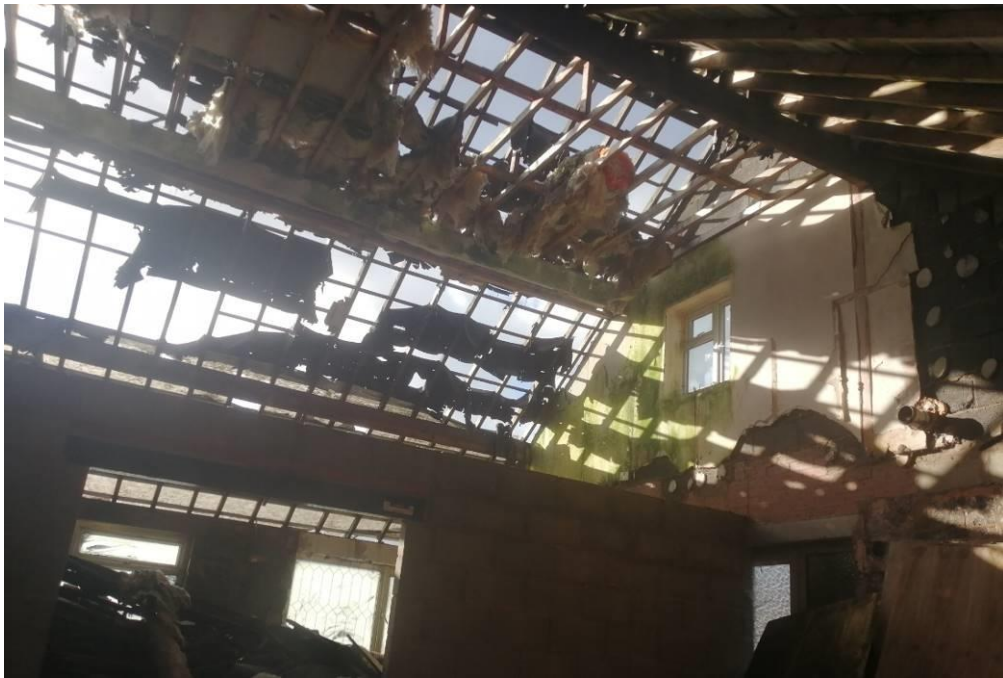
Plate 5- Interior of 119 Cornwall Drive
