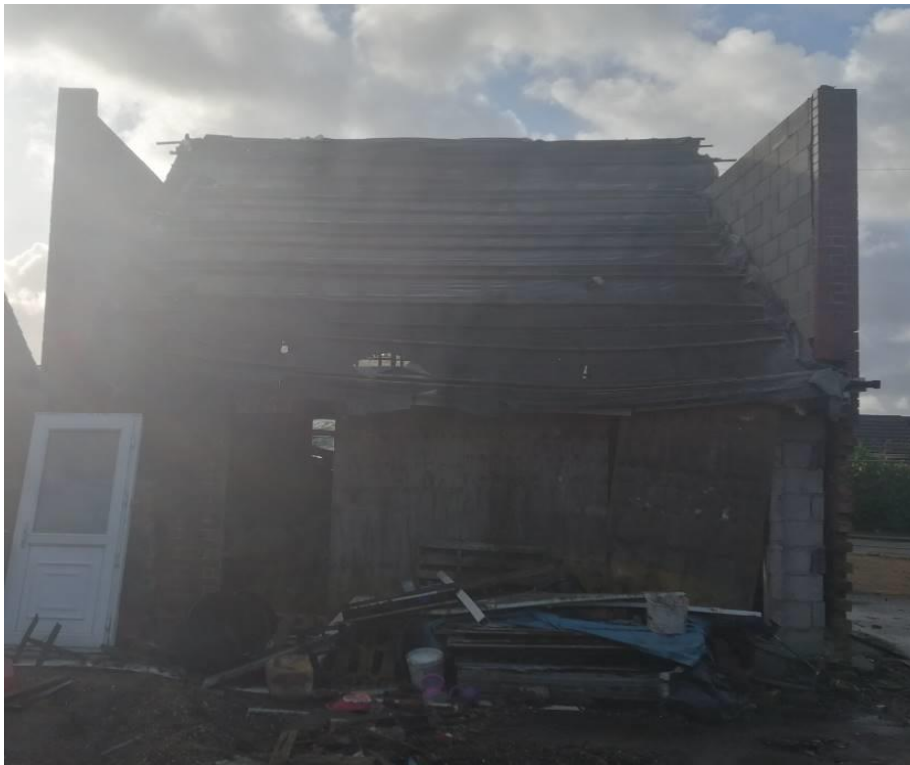
Plate 3- Open (north facing) elevation of 119 Cornwall Drive
