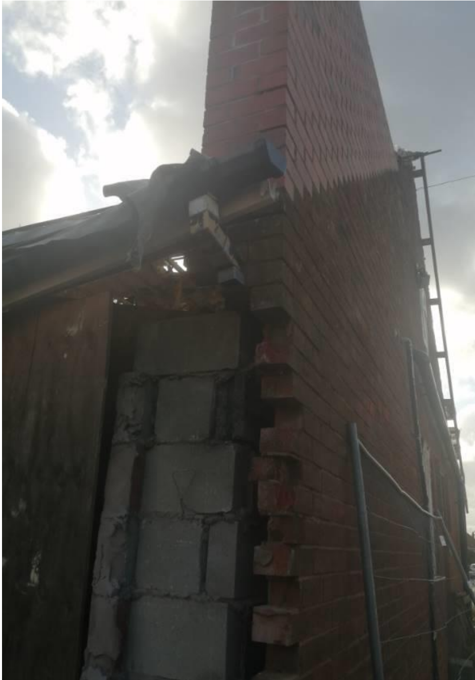
Plate 7- Cavity at 119 Cornwall Drive
