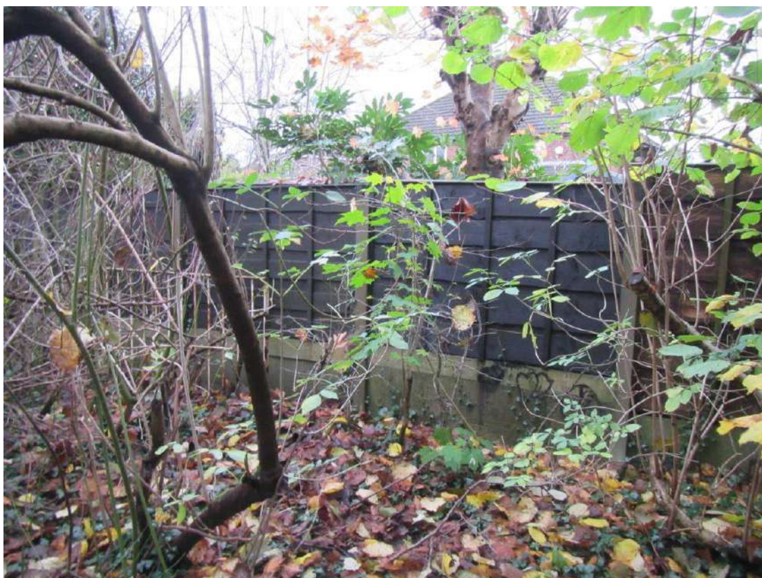
Photograph 7 – Fencing along northern site boundary.
