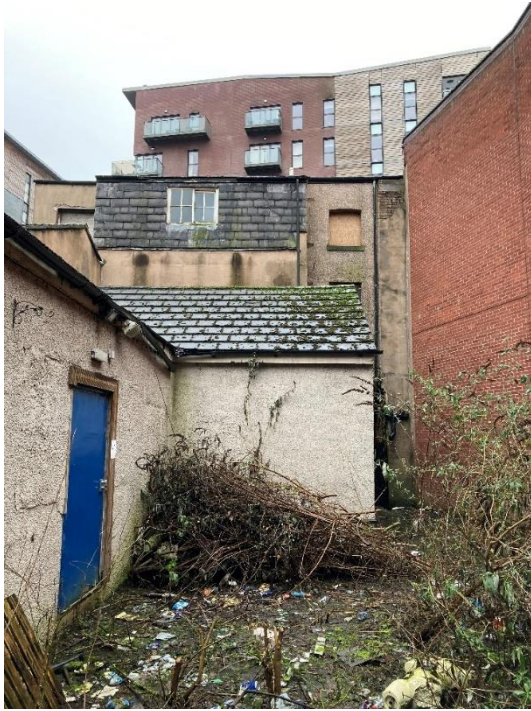
Photograph 2 – Hardstanding courtyard with buddleja growth
