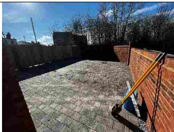
View of rear garden of Plot 8. Soil area will be turfed.
