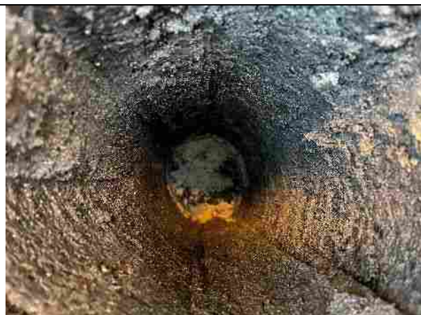
View of soil in capping layer excavation in the northeastern landscaped area. Identified Geo-membrane at base.
