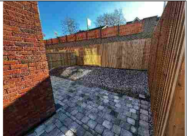
View of rear garden of Plot 6. Retaining wall concrete extends to permeable paving and first generation quarried limestone and gritstone (purchased as a product) present in the photograph will have artificial grass.
