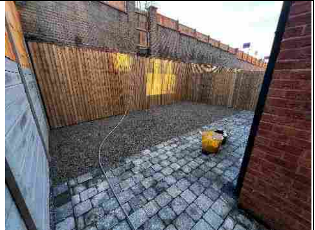
View of rear garden of Plot 1. Retaining wall concrete extends to permeable paving and first generation quarried limestone and gritstone (purchased as a product) will have artificial grass.
