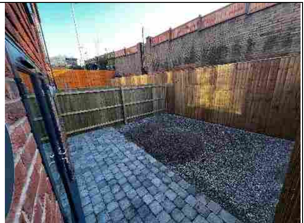
View of rear garden of Plot 2. Retaining wall concrete extends to permeable paving and first generation quarried limestone and gritstone (purchased as a product) will have artificial grass.
