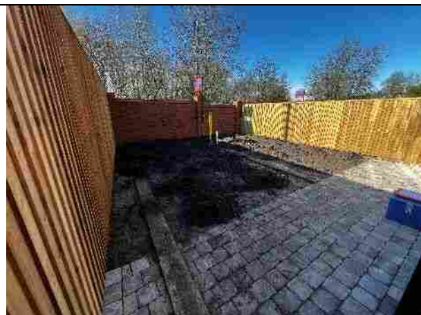
View of rear garden of Plot 7. Soil area will be turfed.
