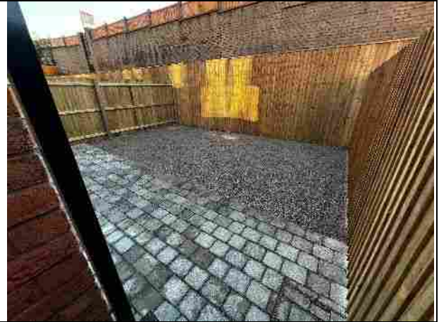
View of rear garden of Plot 3. Retaining wall concrete extends to permeable paving and first generation quarried limestone and gritstone (purchased as a product) present in the photograph will have artificial grass.
