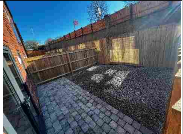
View of rear garden of Plot 5. Retaining wall concrete extends to permeable paving and first generation quarried limestone and gritstone (purchased as a product) present in the photograph will have artificial grass.
