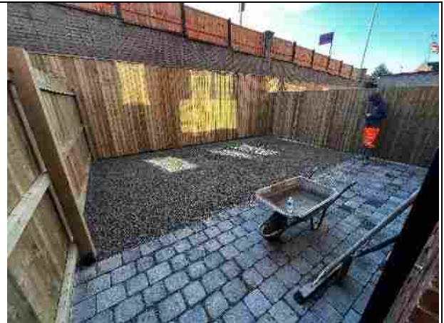
View of rear garden of Plot 4. Retaining wall concrete extends to permeable paving and first generation quarried limestone and gritstone (purchased as a product) present in the photograph will have artificial grass.
