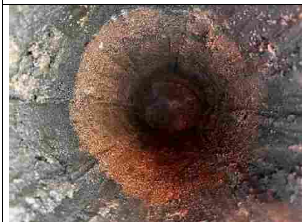
View of soil in capping layer excavation in the rear of Plot 7. Identified Geo-membrane at base.
