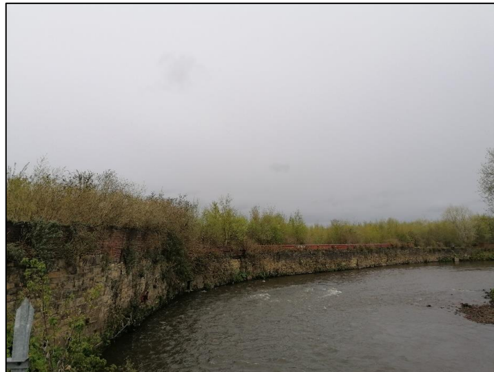
Figure 5 – View of Existing Wall from Crow Trees Farm Brook outfall
