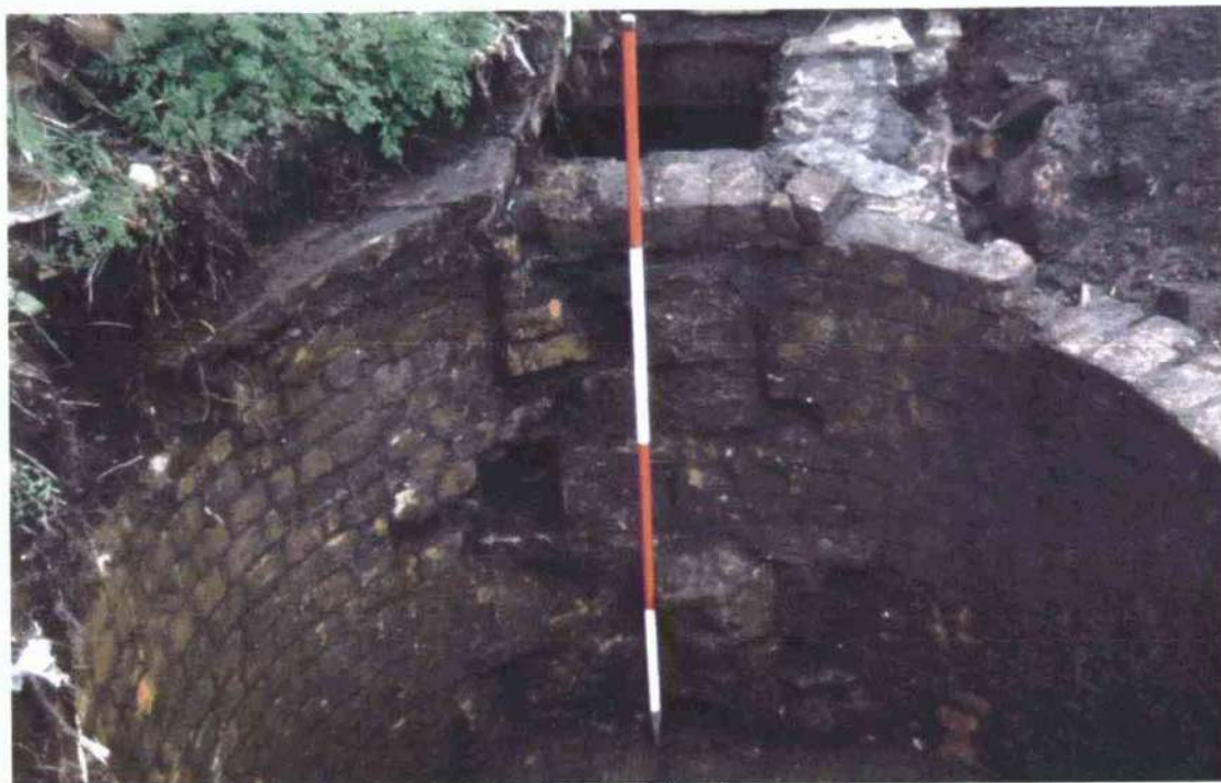
Plate 7: Repair within inner face of chamber 104
