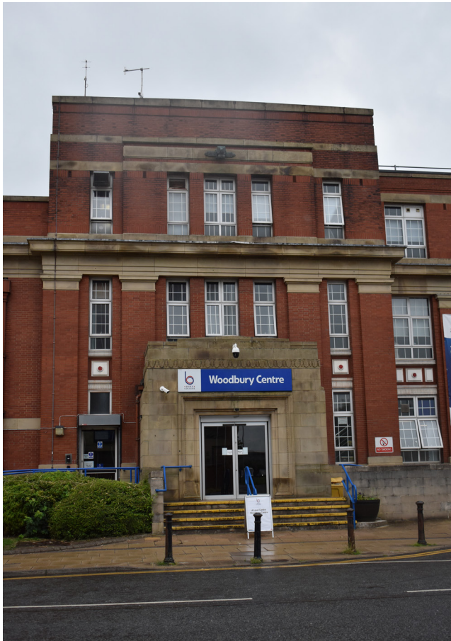
3.42 East Wing, east elevation, south entrance portico
