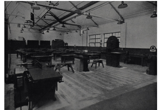
2.26 Carpentry and Joinery Workshop, 1947 (Bury Archives)
