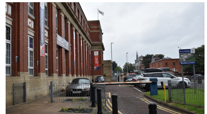
3.25 East car park and access road
