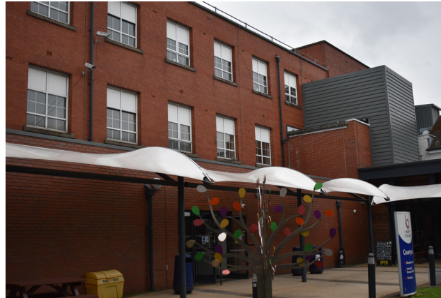
3.63 East Wing, west elevation (north), single-storey projection and modern insertions
