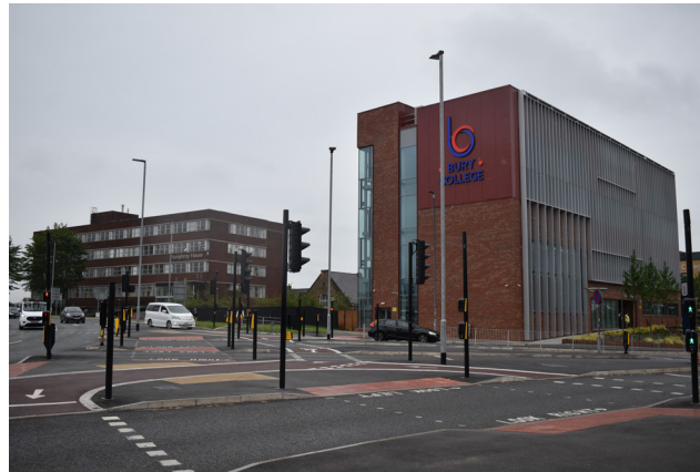
3.2 Angouleme Way, junction with Market Street, looking east
