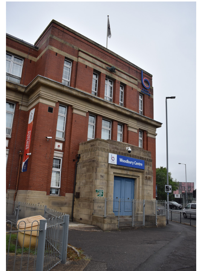
3.41 North Wing, east elevation, north pavilion and entrance portico
