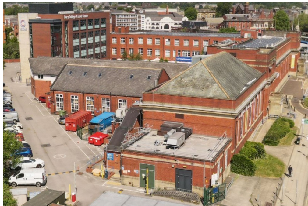
3.64 Woodbury Centre roofs, c.2021 (Bury College)
