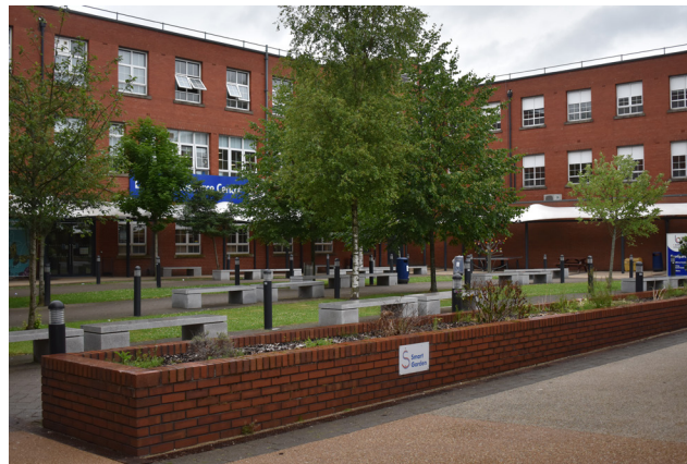
3.59 North Wing south elevation and East Wing west elevation, viewed from the courtyard
