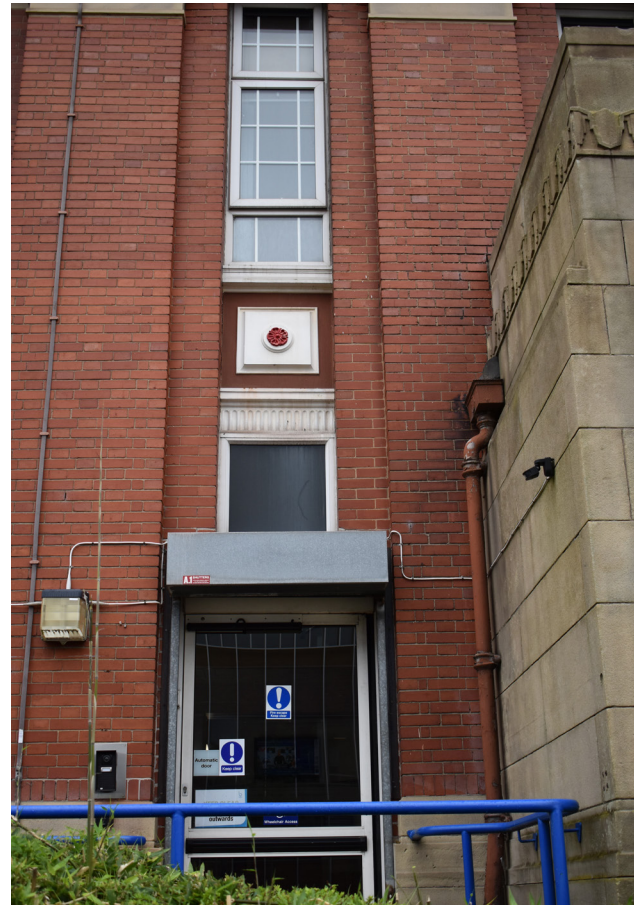
3.43 East Wing, east elevation, altered fenestration to the south of the south entrance portico to provide wheelchair access
