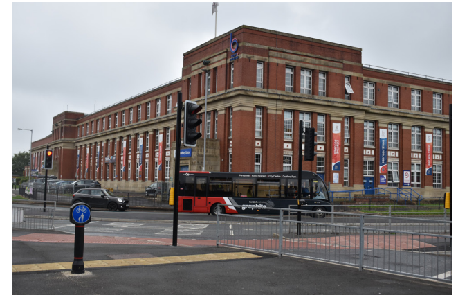
3.4 Complex crossings to the east and north, with a multiplicity of street furniture
