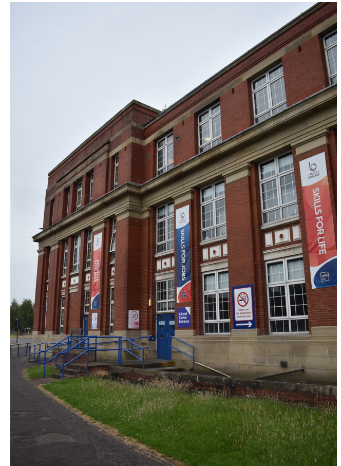
3.49 North elevation, projecting north pavilion
