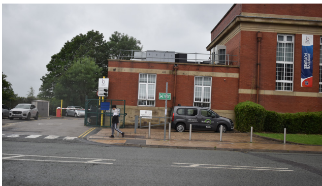
3.30 Service road entrance into the rear
