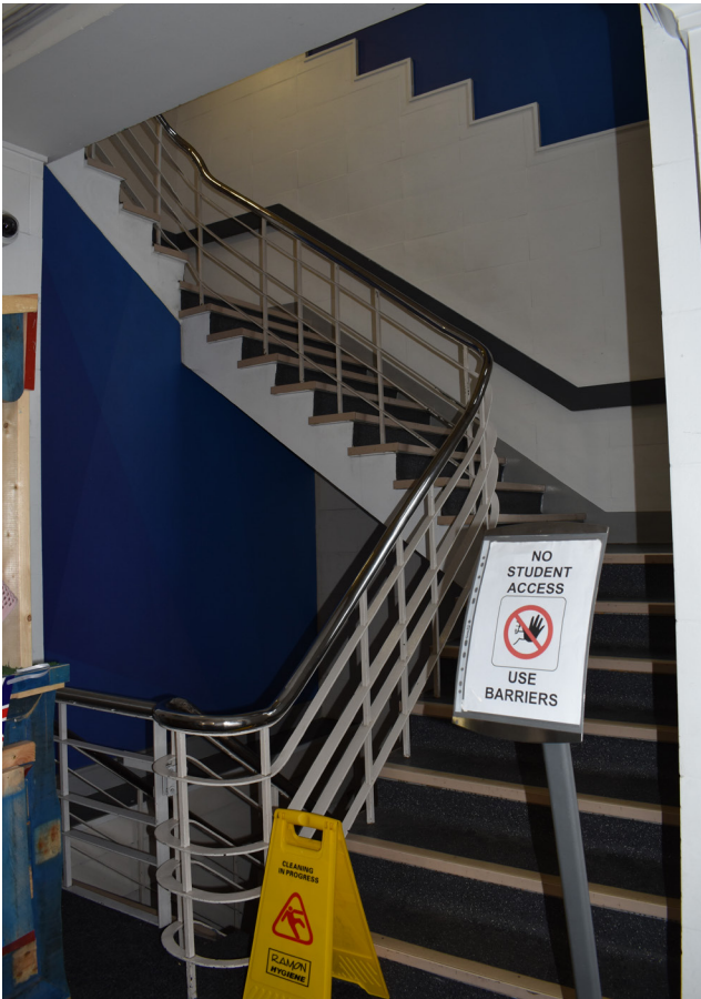
3.75 South entrance stairs
