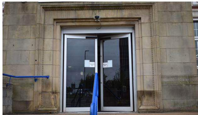
3.44 East Wing, east elevation, modern doors in the south entrance portico
