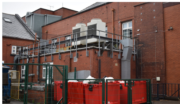
3.52 East Wing, rear (west), single-storey structure
