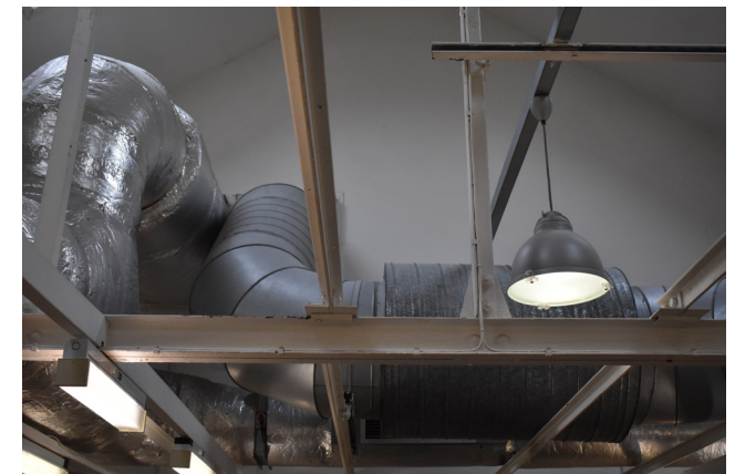
3.80 Former Gymnasium, ducting
