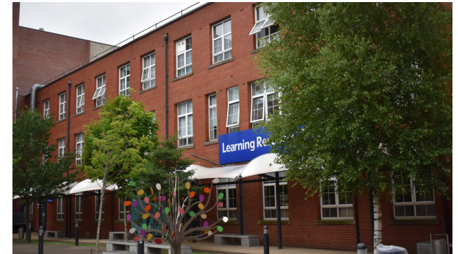
3.60 North Wing, south elevation, looking west
