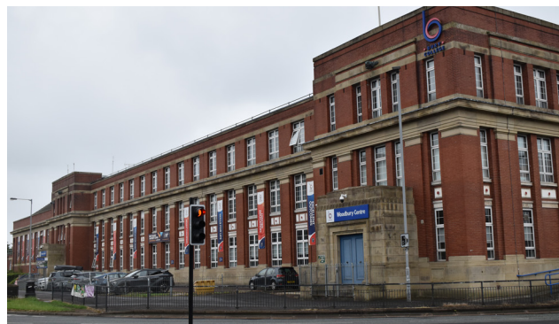
3.23 North pavilion (with entrance portico) and truncated east drive
