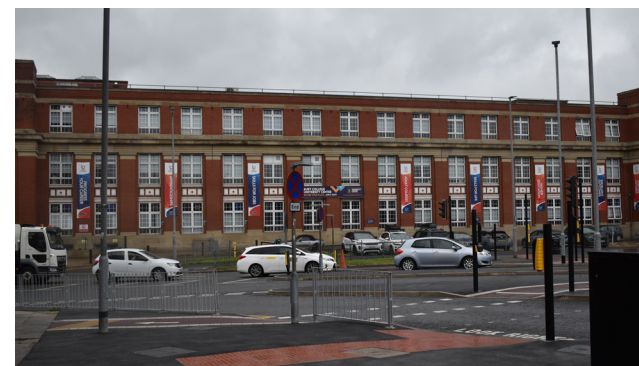
3.39 East Wing, east elevation, main range
