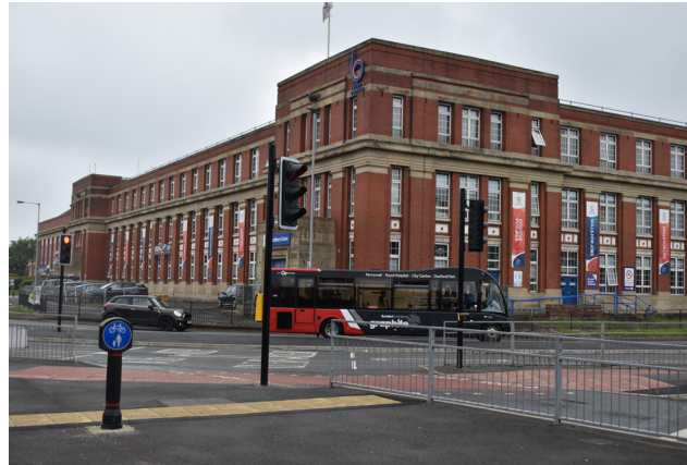
3.4 Complex crossings to the east and north, with a multiplicity of street furniture
