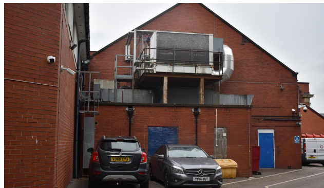
3.55 (Former) Gymnasium, west elevation
