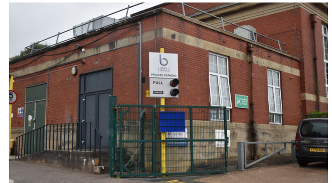
3.47 East Wing, substation building, east (R) and south (L) elevations
