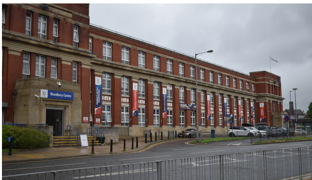
3.27 East car park
