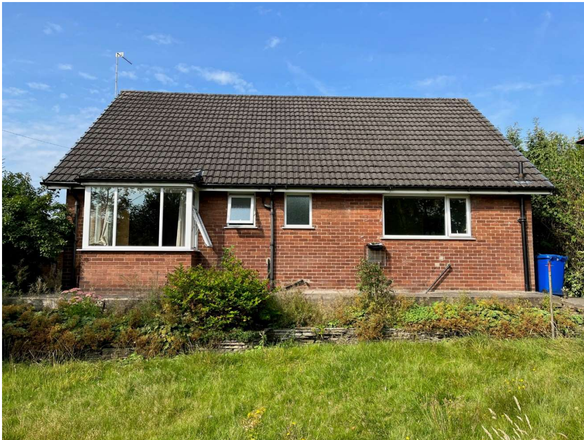
Photo 2 – Rear view of the existing property
