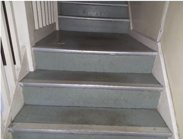
Sample No: 22/12/B/13/MAC10 G.02 Rear of shop Stairs Vinyl floor covering No Asbestos Detected
