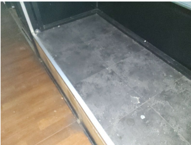
Sample No: 22/12/B/13/MAC5 G.01 Front of shop Front window display floor Vinyl floor tiles No Asbestos Detected
