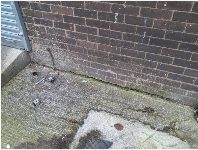
Sample No: 22/12/B/13/MAC14 External Walls Bitumen DPC No Asbestos Detected
