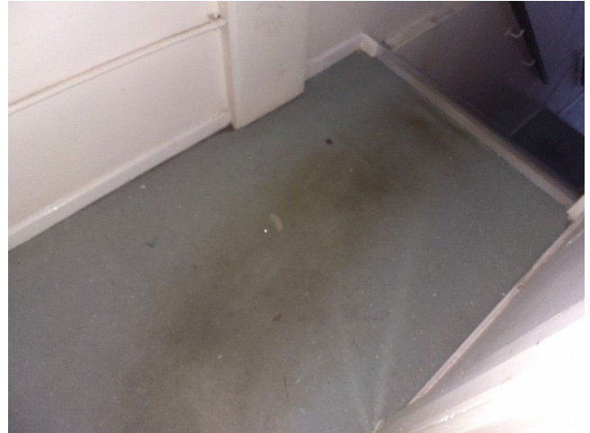
Sample No: Refer to Sample 22/12/B/13/MAC10 1.03 Landing Stairs Vinyl floor covering No Asbestos Detected
