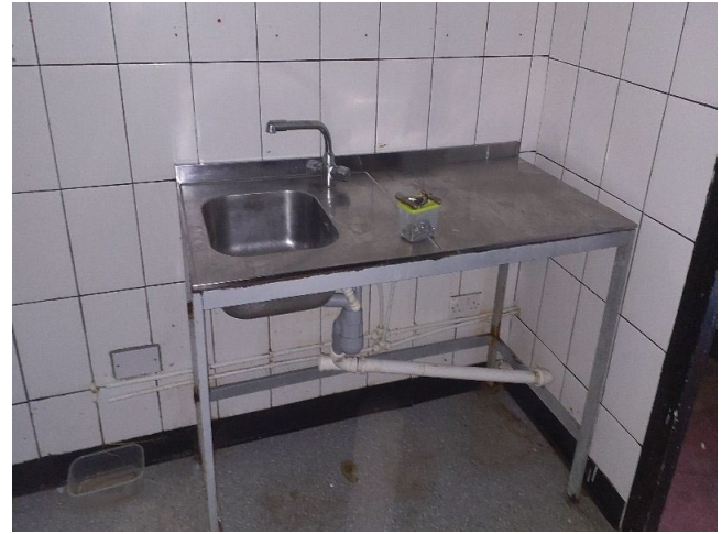
Sample No: 22/12/B/13/DAB15 G.03 Kitchen Sink Bitumen sink pad No Asbestos Detected
