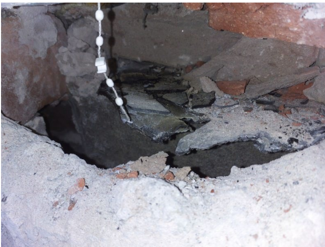
Sample No: Refer to Sample 22/12/B/12/SAW4 External Windows Bitumen vapour barrier to wall cavities No Asbestos Detected
