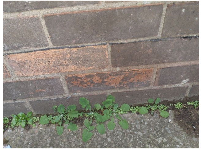
Sample No: 22/12/B/12/SAW5 External Damp proof course Bitumen Layer No Asbestos Detected
