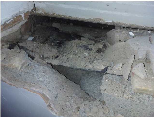
Sample No: Refer to Sample 22/12/B/12/SAW9 External Windows Bitumen vapour barrier to wall cavities No Asbestos Detected
