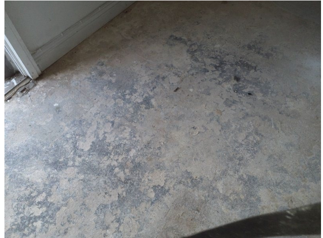
Sample No: Refer to Sample 22/12/B/12/SAW6 G.04 Circulation area Floor beneath screed Bitumen residuals containing: Chrysotile
