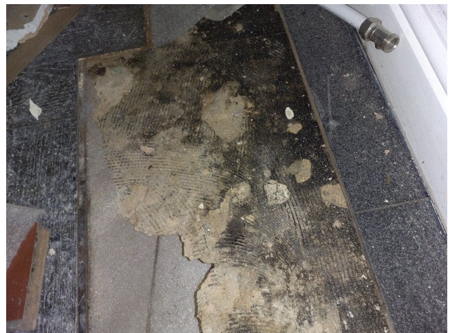
Sample No: Refer to Sample 22/12/B/12/SAW6 G.06 Toilet Floor Bitumen residuals containing: Chrysotile
