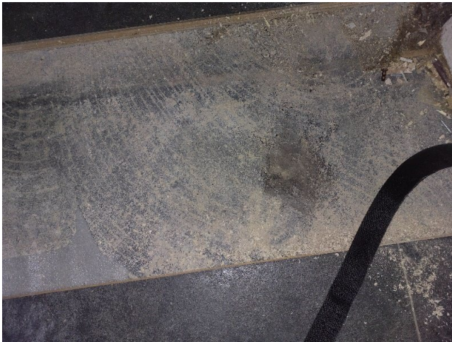
Sample No: 22/12/B/12/SAW7 1.01 Landing Floor Bitumen residuals containing: Chrysotile
