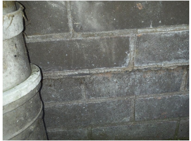
Sample No: 22/12/B/12/SAW10 External Damp proof course Bitumen Layer No Asbestos Detected
