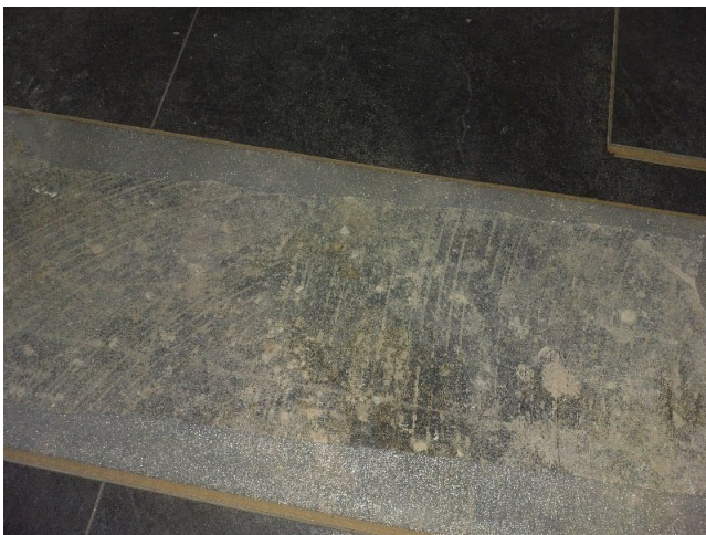
Sample No: Refer to Sample 22/12/B/12/SAW7 1.03 Circulation Floor Bitumen residuals containing: Chrysotile
