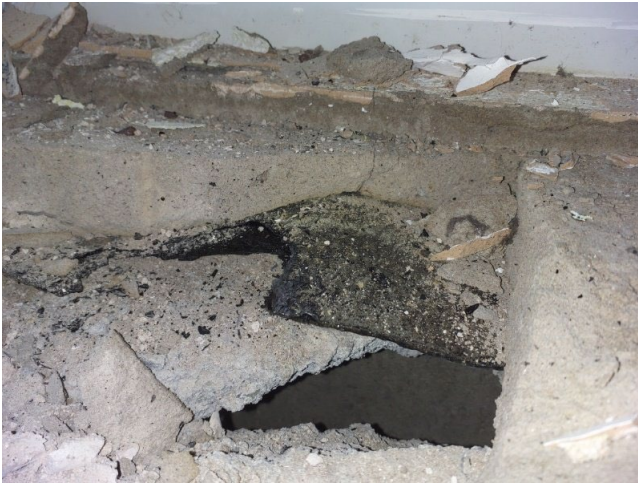
Sample No: 22/12/B/12/SAW9 External Windows Bitumen vapour barrier to wall cavities No Asbestos Detected
