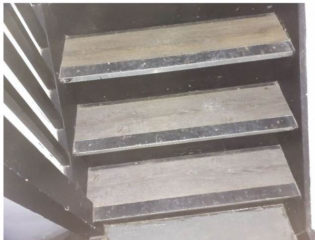
Sample No: 22/12/B/12/SAW8 1.07 Stairs Staircase Nose edging No Asbestos Detected
