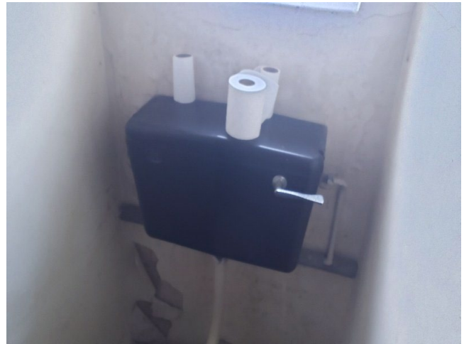
Sample No: Refer to Sample 22/12/B/12/MBK8 2.05 Ladies toilet Toilet Cistern Thermoplastic containing: Amosite
