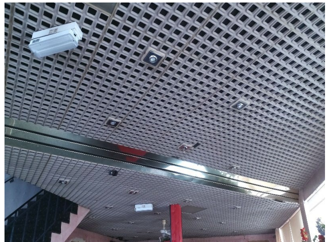
Sample No: 22/12/B/12/MBK2 G.01 Main shop floor Ceiling Suspended insulation tiles No Asbestos Detected
