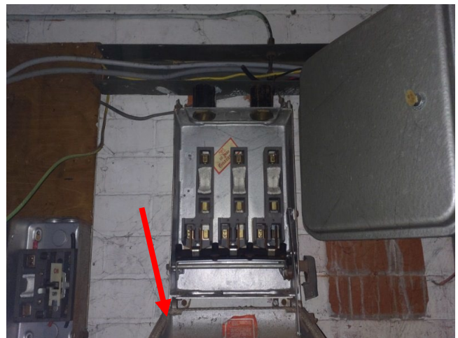
Sample No: 22/12/B/12/MBK12 B.01 Store room / Electrics room Fuse boxes Woven rope seal No Asbestos Detected
