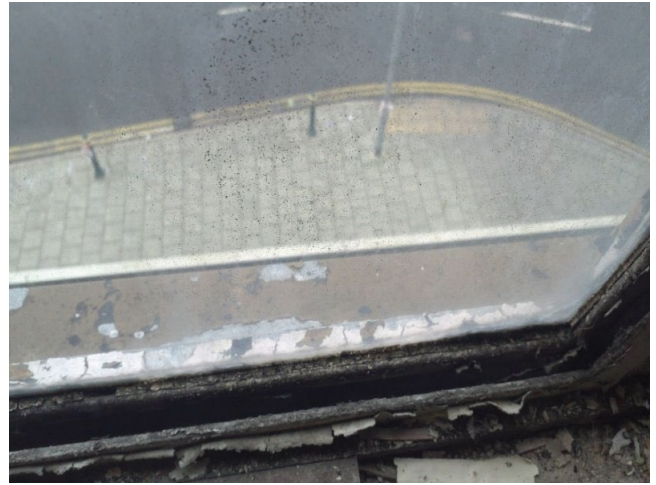
Sample No: 22/12/B/12/MBK11 External Metal windows Putty No Asbestos Detected
