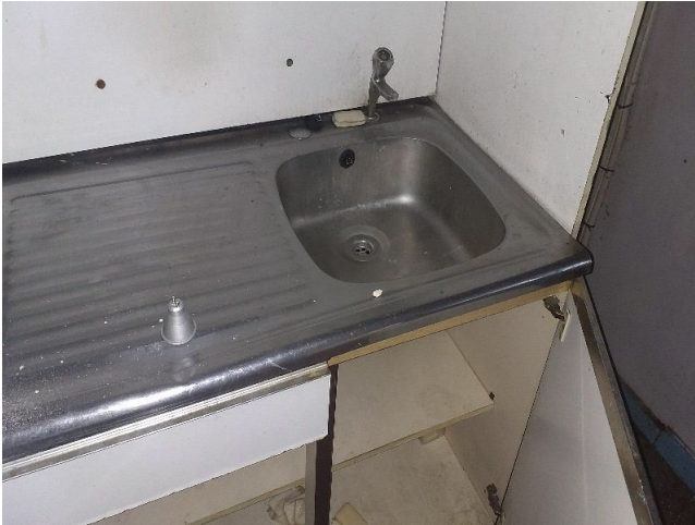
Sample No: 22/12/B/12/MBK3 G.02 Kitchen Sink Bitumen pad No Asbestos Detected
