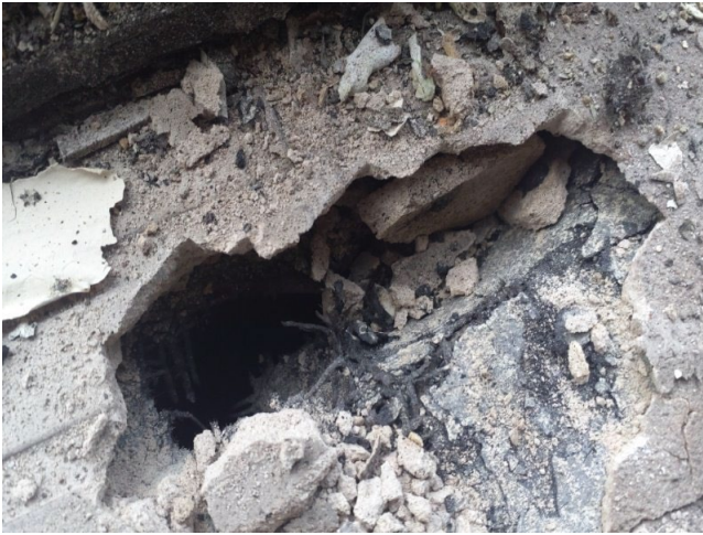
Sample No: 22/12/B/12/MBK10 External External walls Bitumen damp barrier felt No Asbestos Detected
