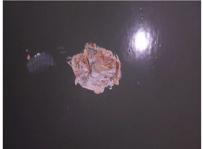
Sample No: 22/12/B/12/MBK6 1.01 Stairs / Landing Double fire door internal lining Insulation board No Asbestos Detected
