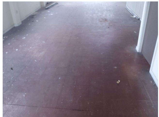
Sample No: 22/12/B/12/MBK7 2.01 Open plan storage space Floor Vinyl Floor Tiles and Bitumen Adhesive containing: Chrysotile (In both tile and bitumen)
