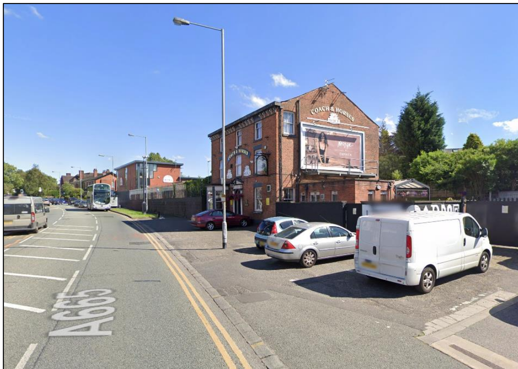
Figure 2b: Street level view of site (Western Elevation)
