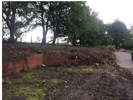
Photograph 3 (P3) Raised area along the north of the site. Bricked wall acting as retaining feature.
