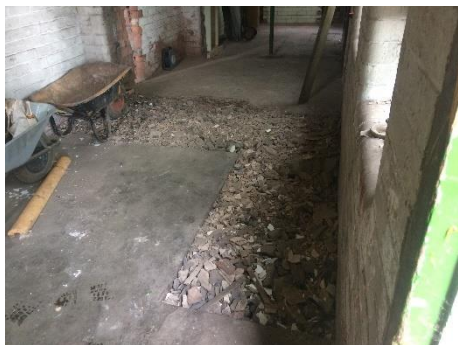
Photograph 8 (P8) Inside 'Wash House' where former coal burner was below ground level.
