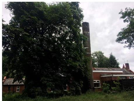
Photograph 9 (P9) Chimney in the east of site next to mature tree.
