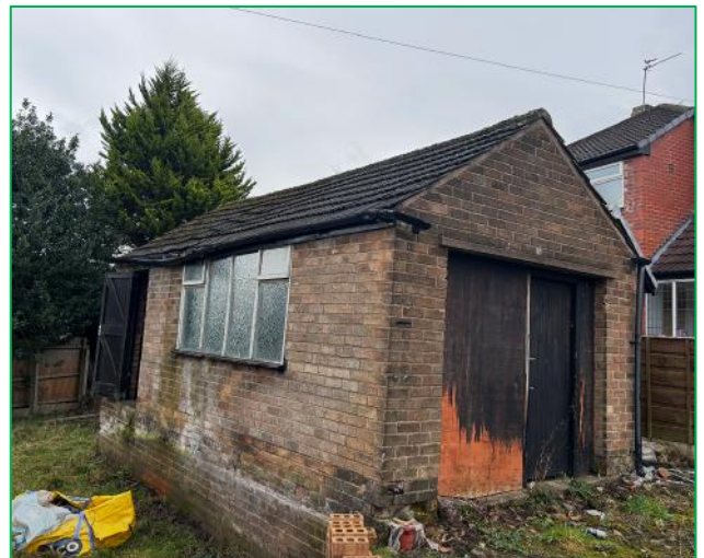
The west and north elevation of the shed
