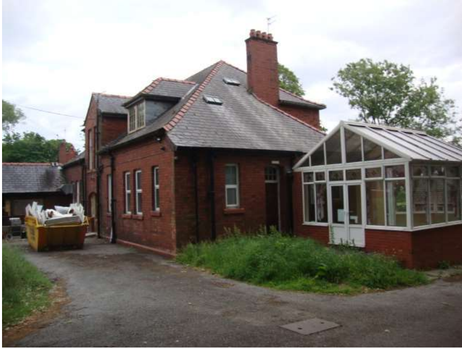
Figure 2 – Rear elevation to Administration Block
