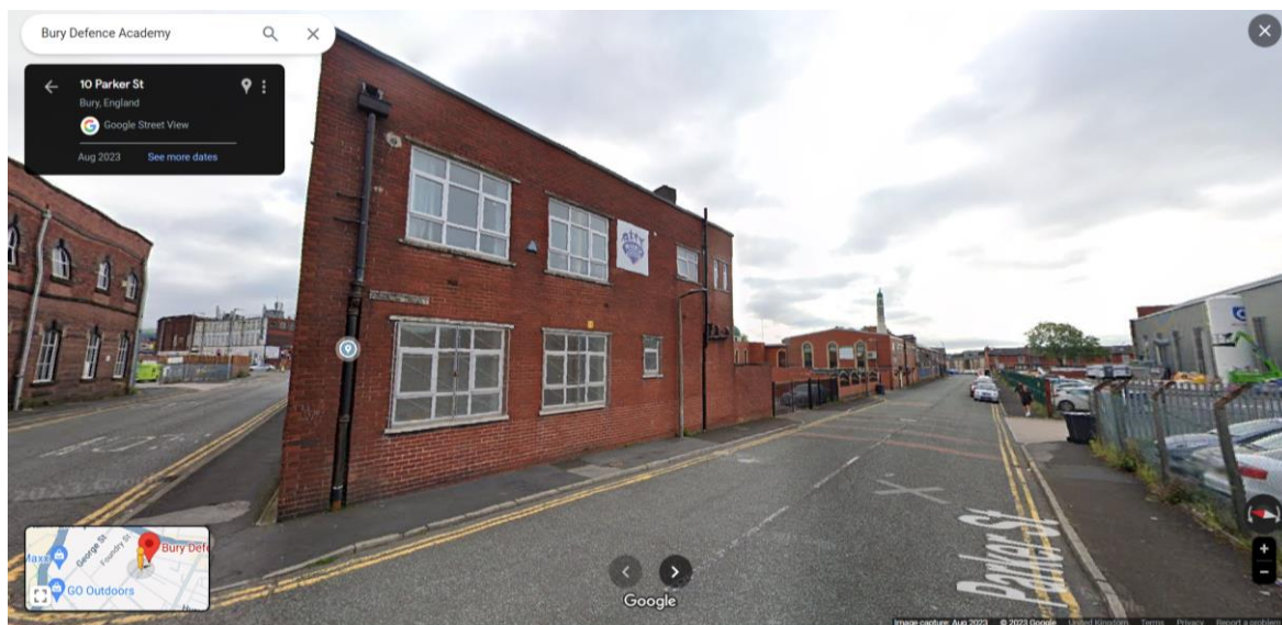
Image Courtesy of Google Photo 3 The building from Parker Street
