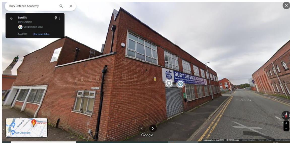
Image courtesy of Google Photo 2 The building from Lord Street
