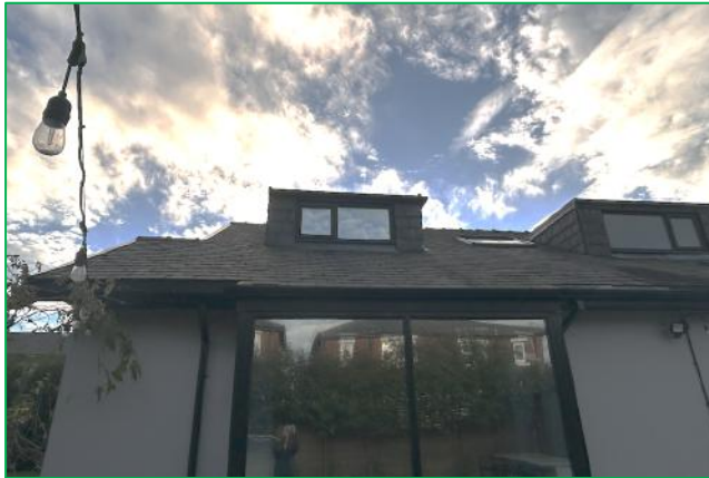
The rear (north elevation) of the house
