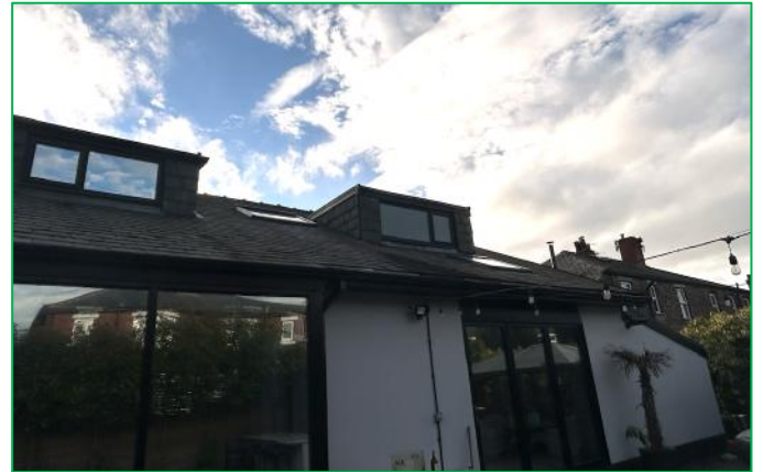
The rear (north elevation) of the house
