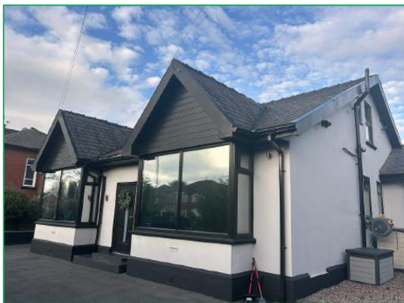
The front (south elevation) of the house
