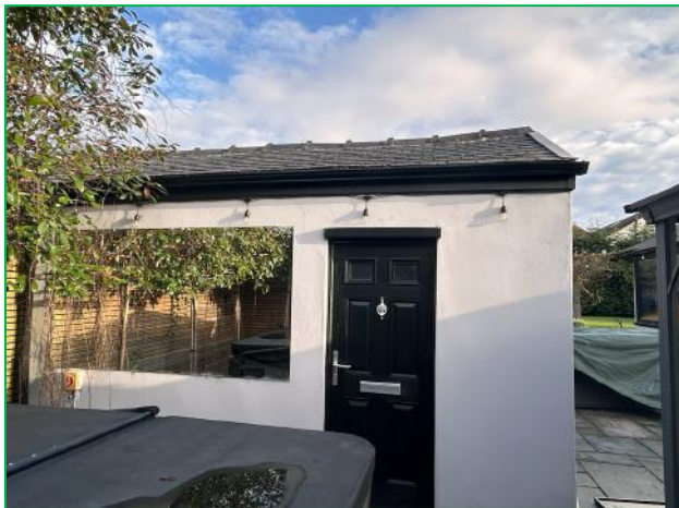
The west elevation of the shed
