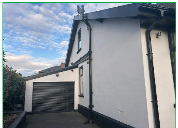
The front (south elevation) of the house
