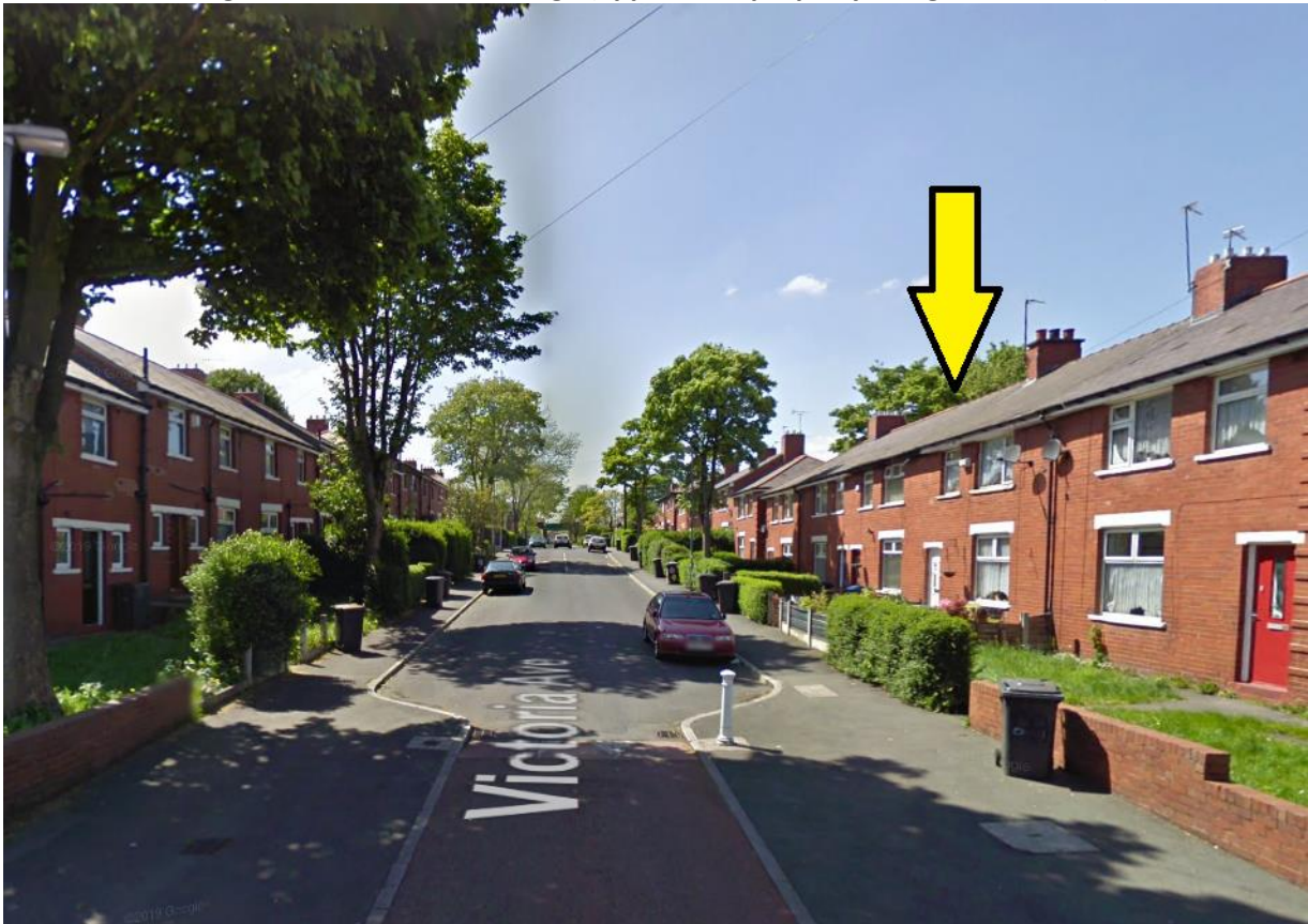
Figure 6 – Street scene image (application property to right hand side)
