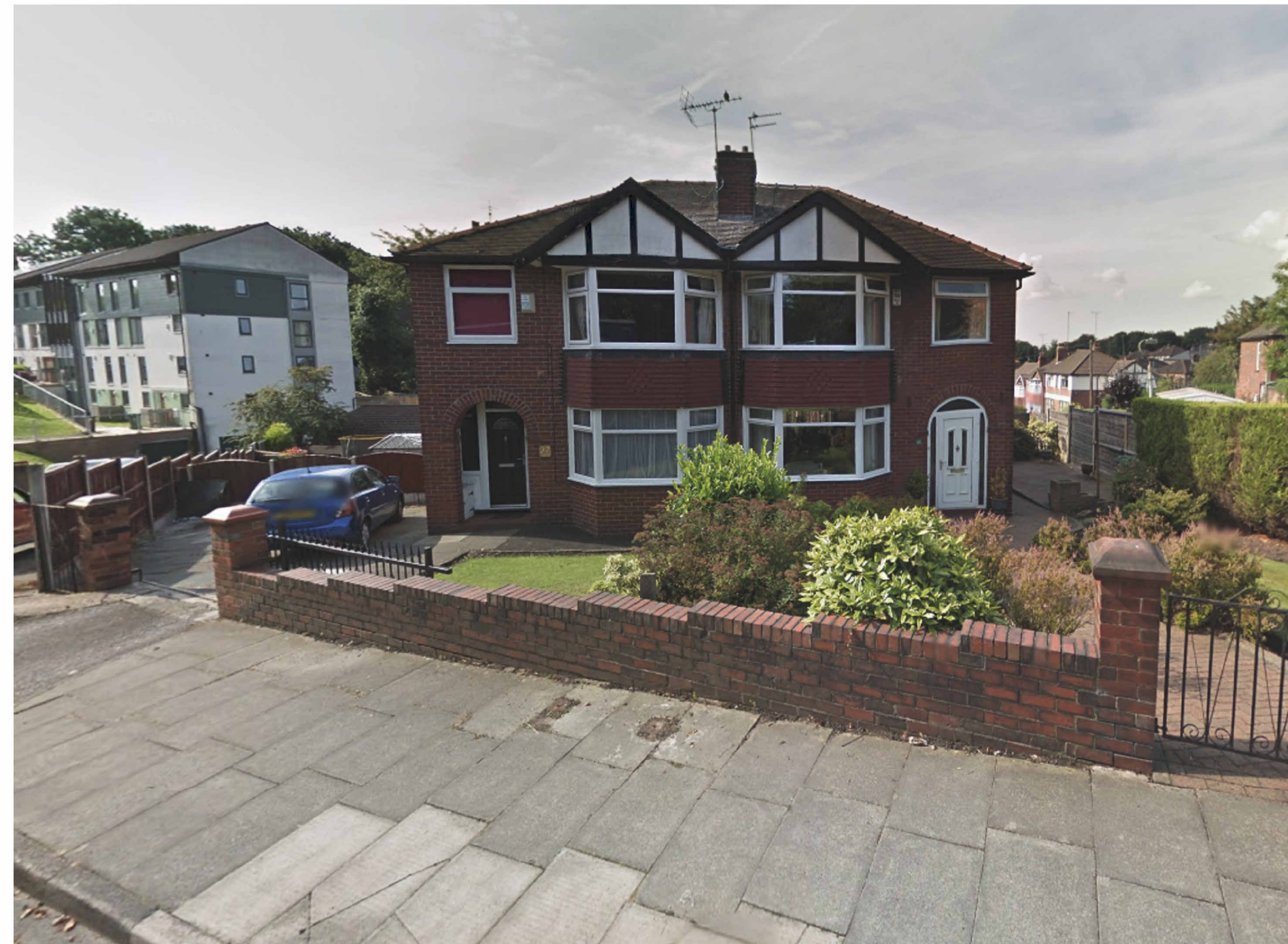
Street Scene - 22 Church Drive
