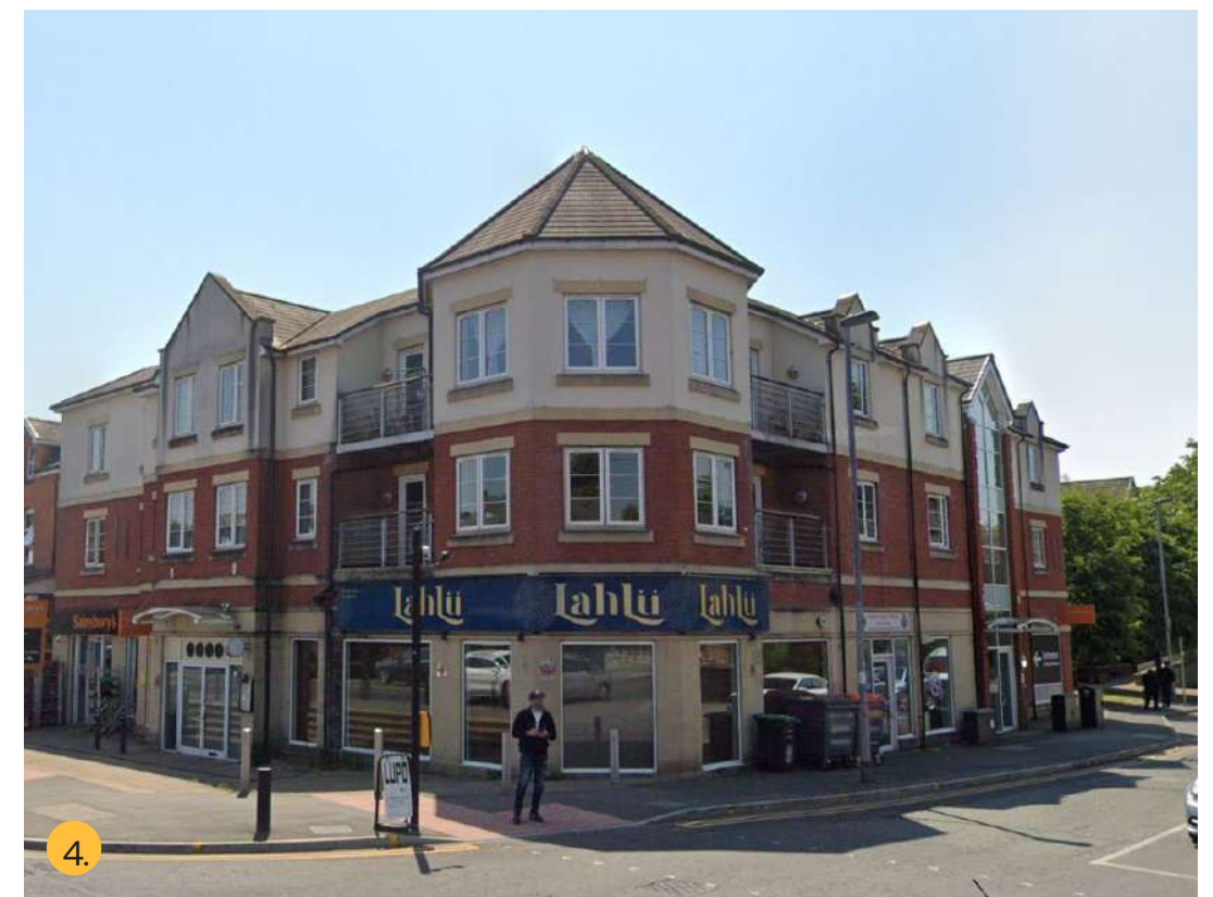
3 storey apartment block on George St/Bury New Rd Junction.
