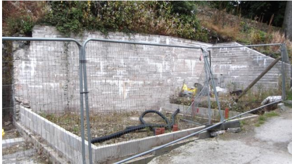
(17) New retaining and flanking wall
