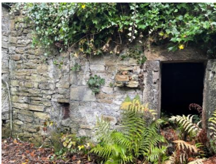
(24) Good quality tooled stone framing
