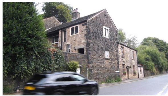
(14) Higher House Cottage/barn and 3 Helmsore Road
