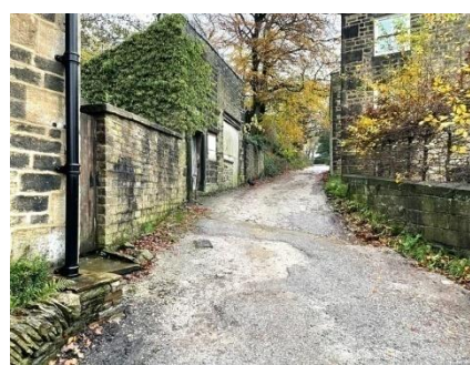
(22) Moor Road, watershot wall and gate
