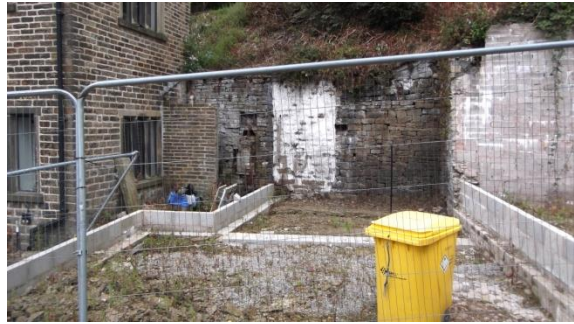
(16) Original stone retaining wall
