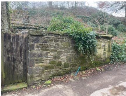
(21) Boundary wall in north
