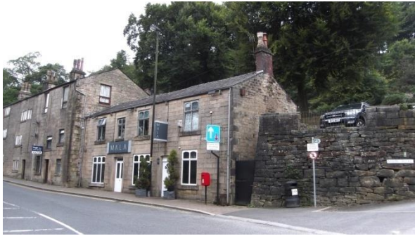
(13) 18 to 34 Holcombe Village
