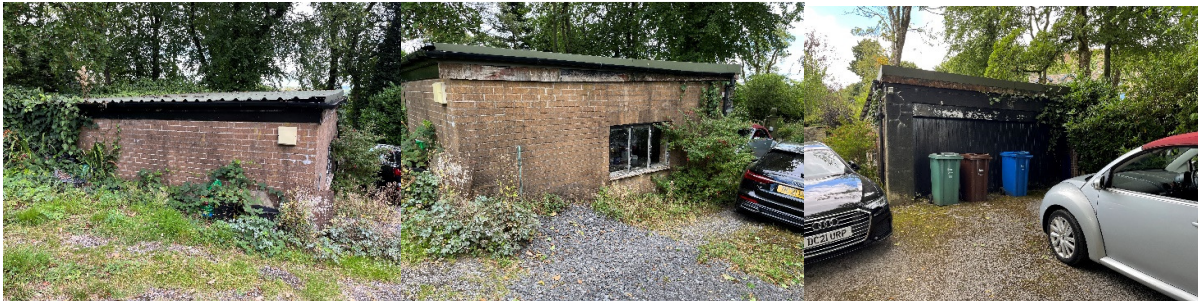
Existing Garage Rear Elevation
