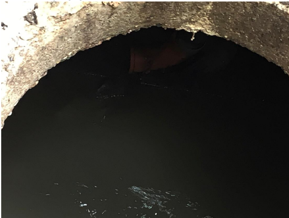
Photo of MH 4702 with evidence of 150mm dia plastic pipe former site connection on far side of channel. Flow going right to left.
