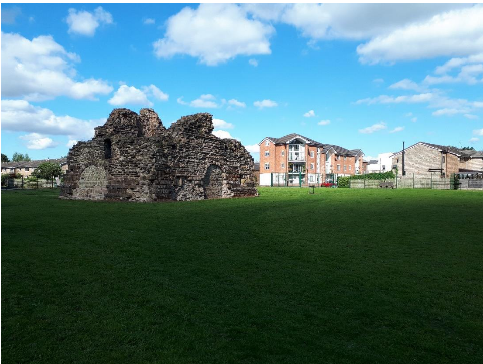
Photo 2: Radcliffe Tower. Facing North-west
