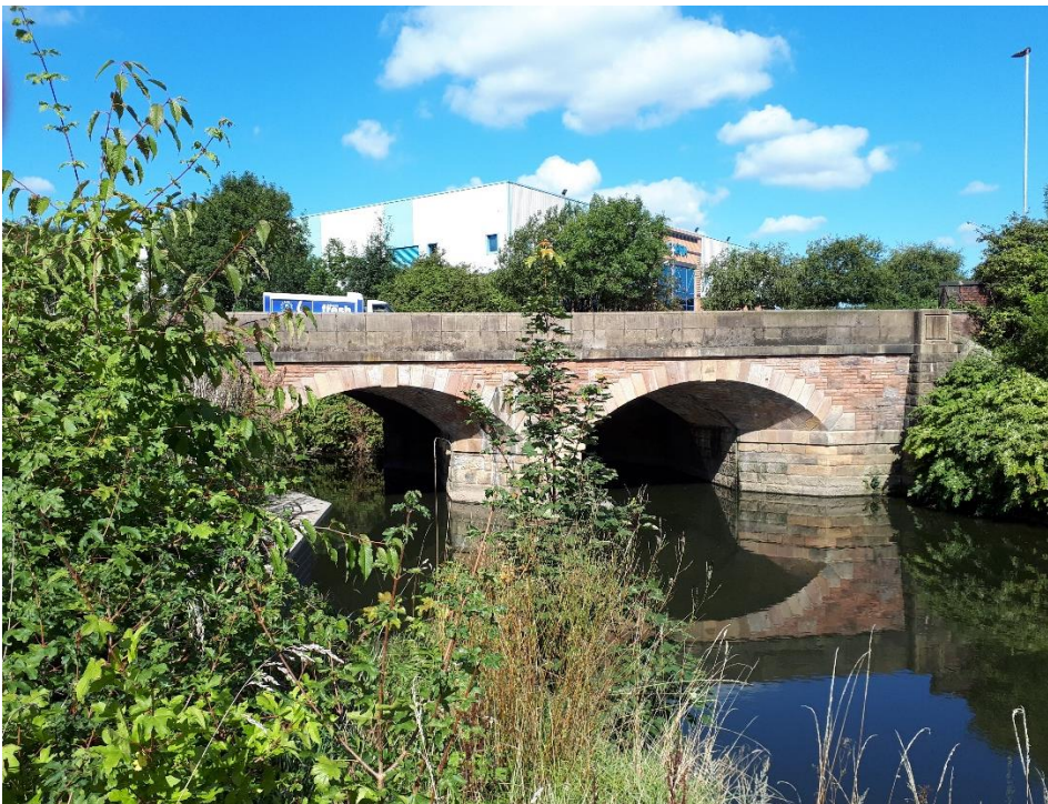
Photo 5: Hardy's Gate Bridge from Riverside Walk. Facing North-west
