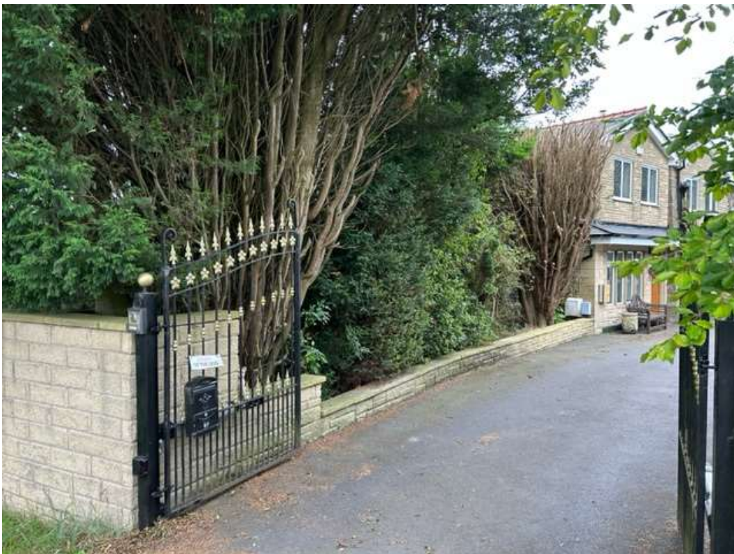
Plate 4 – Adjacent gate and walling to Titus Cottage
