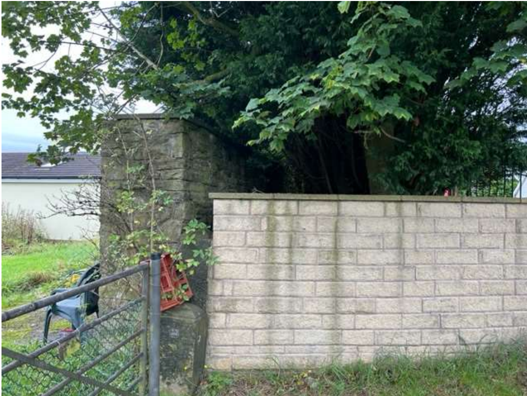
Plate 3 – Existing gate and walling at site access
