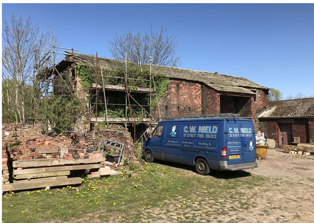
view of two storey barn
