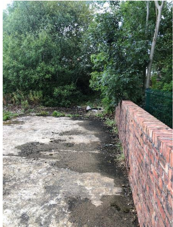
Photograph 7: Wall and security fence along riparian corridor providing barrier between the site and brook.
