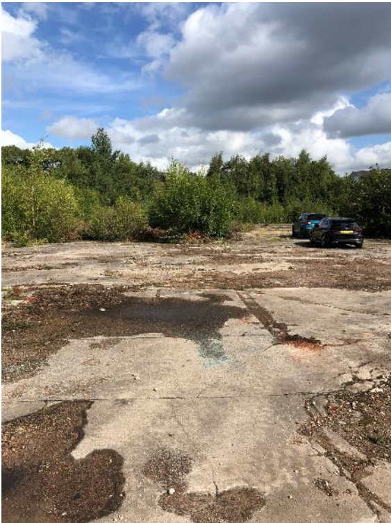
Photograph 1: Overview of the site looking north from the southern boundary.
