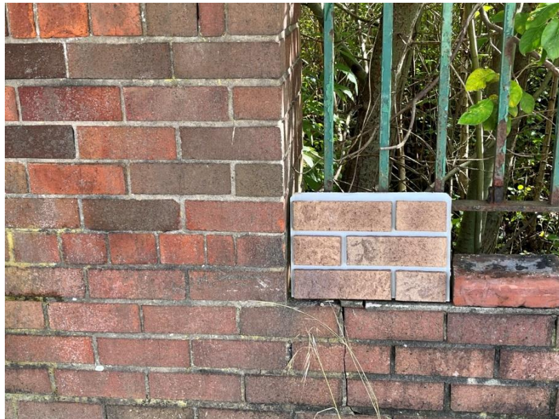
Figure 41 Ibstock Milburn Ashen Brown blend brick sample next to original site boundary wall.
