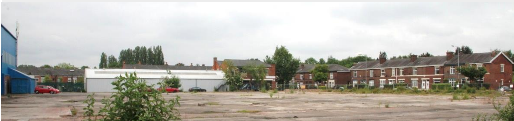
Figure 3 View to south-west of site
