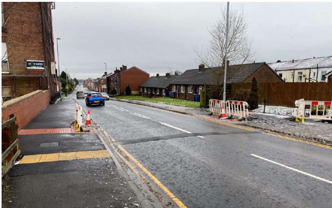
Photograph 2.4 – Higher Ainsworth Road Signalised Crossing (under construction)
