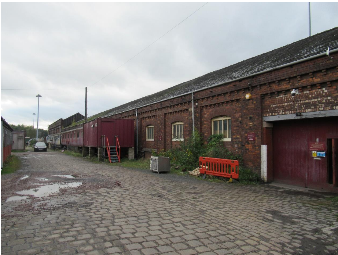
Photograph 2 – The middle section of the south-eastern aspect.
