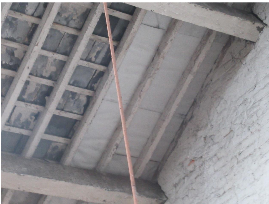
Photograph 16 – Small section of modern breathable roofing membrane in the north-western section.
