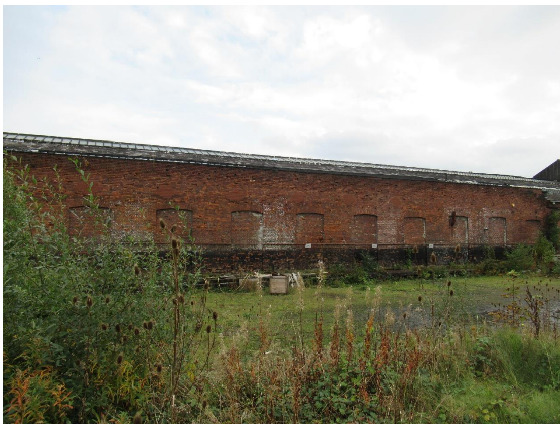
Photograph 6 – The middle section of the north-western aspect.
