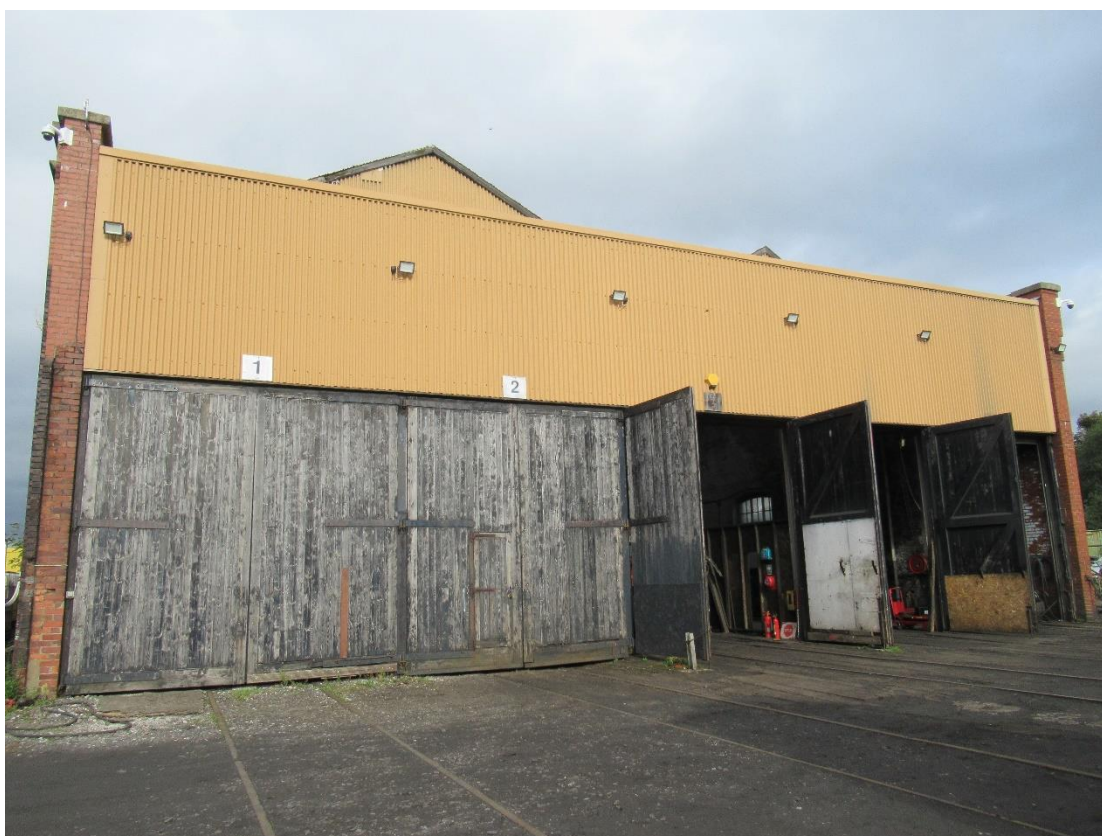
Photograph 4 – The south-western aspect, showing the two-storey extension.
