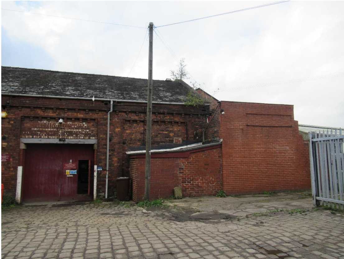
Photograph 1 – The northern section of the south-eastern aspect, showing the single storey extension.
