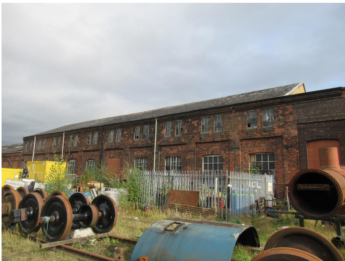
Photograph 5 – The southern section of the north-western aspect.
