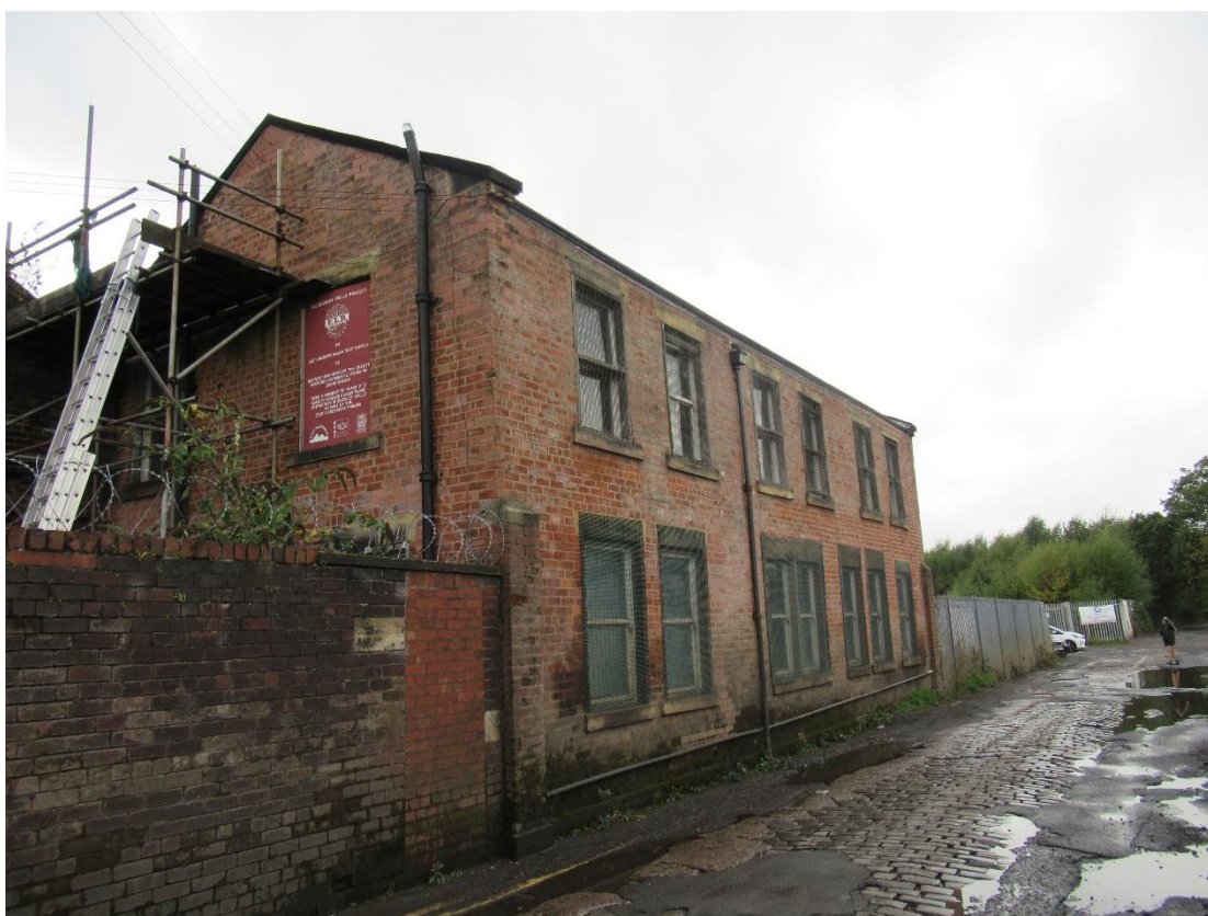
Photograph 8 – The north-eastern aspect, showing the two-storey extension.
