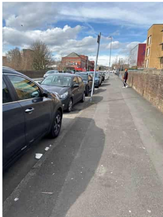
(40) Sign post leaning on southbound footway
