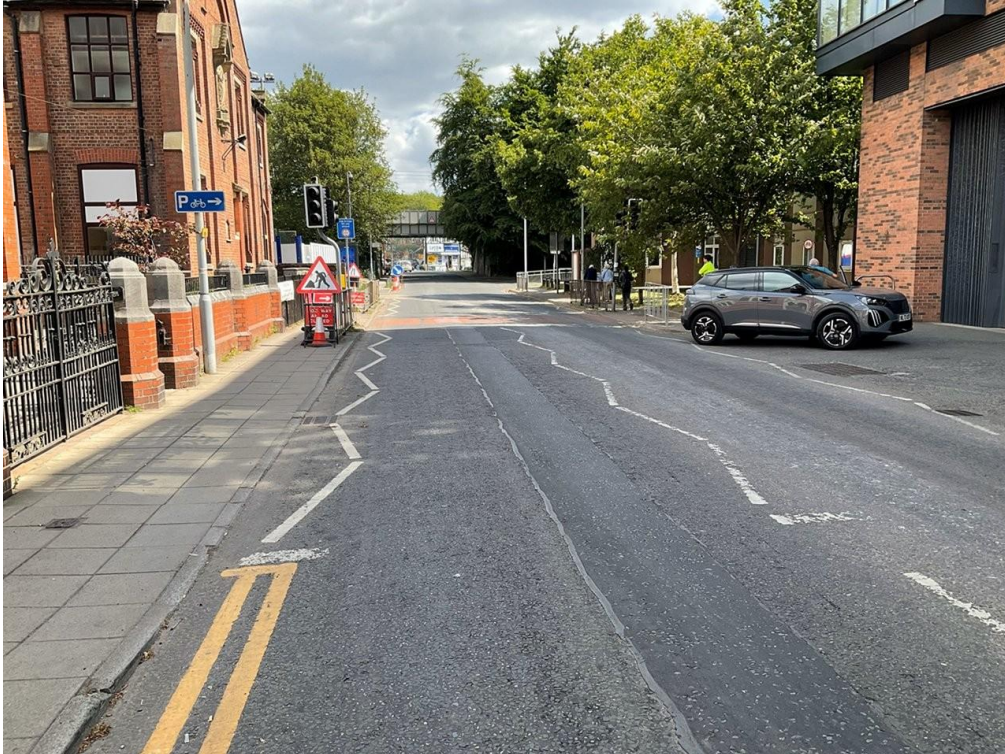
6.1 General view looking east on Fairfax Road towards the proposed junction.
