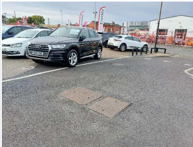
Image 23: Double manhole chamber evident in the centre of the site near the entrance / exit to Bridge St. Tarmac surfacing, sloping down to the western boundary. Facing southwest.
