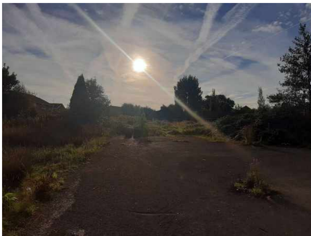
Plate 2 The remains of the access road
