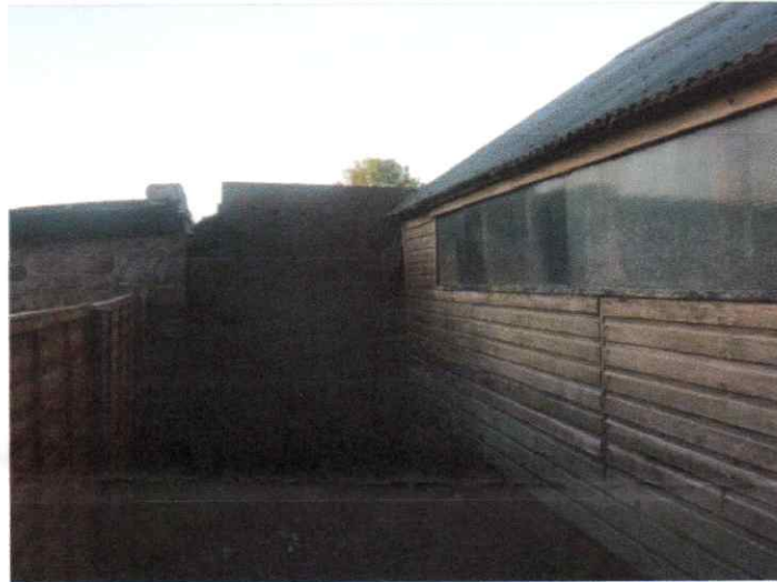
P7 Next door building obstructing rear of affected stables
