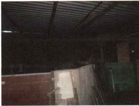
P3 Inside main section, unlined roof
