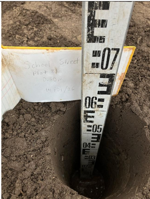
Plot 1: Overview of excavation
