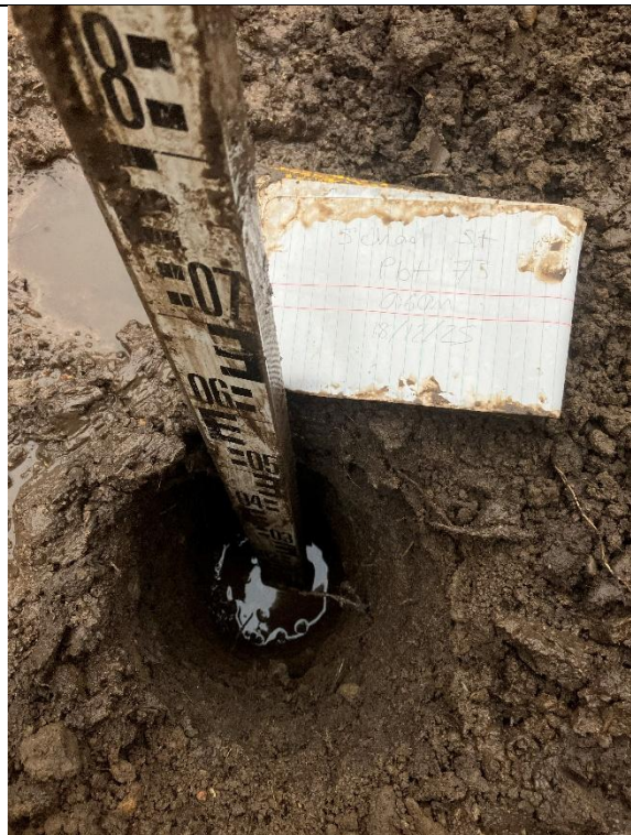
Plot 1: Overview of excavation
