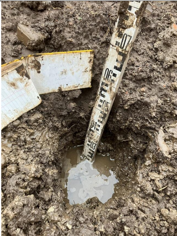
Plot 1: Overview of excavation
