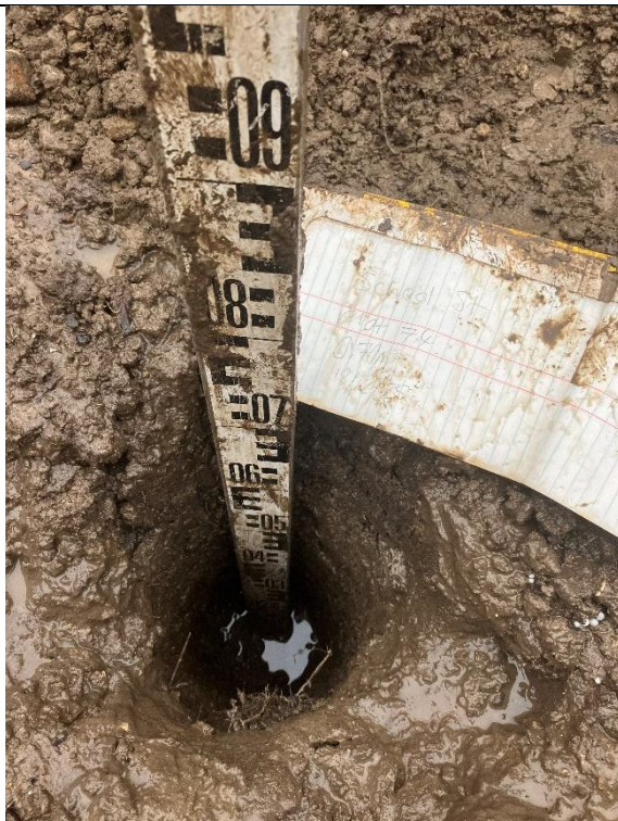
Plot 1: Overview of excavation
