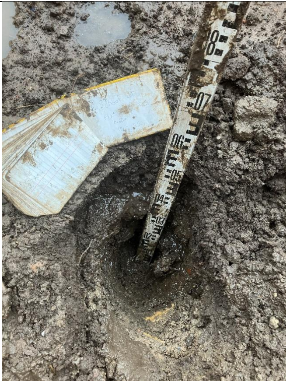
Plot 1: Overview of excavation
