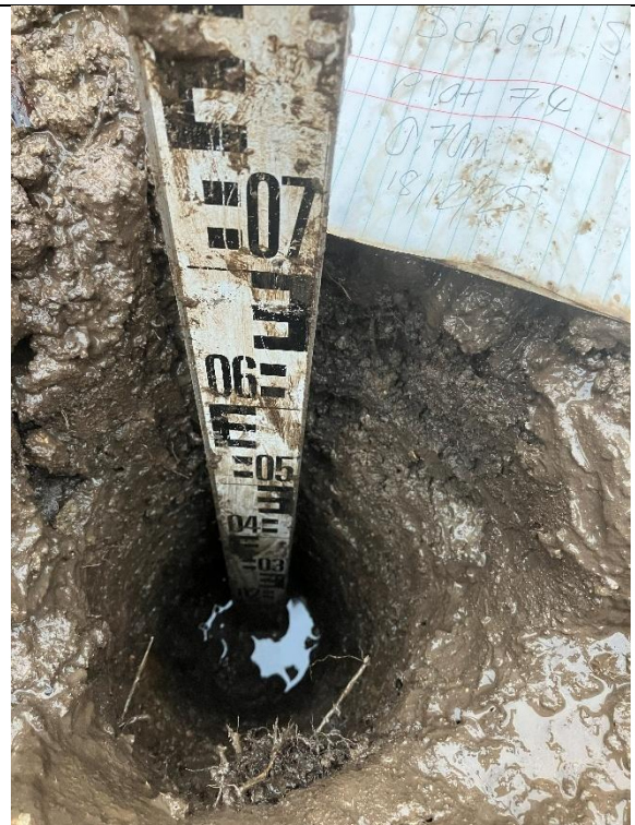
Plot 1: Internal View of excavation
