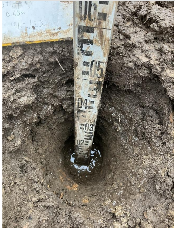
Plot 1: Internal View of excavation
