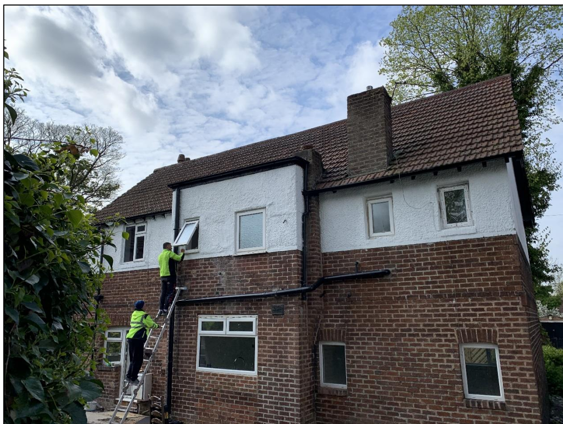
Plate 2 – The north-eastern aspect of the structure
