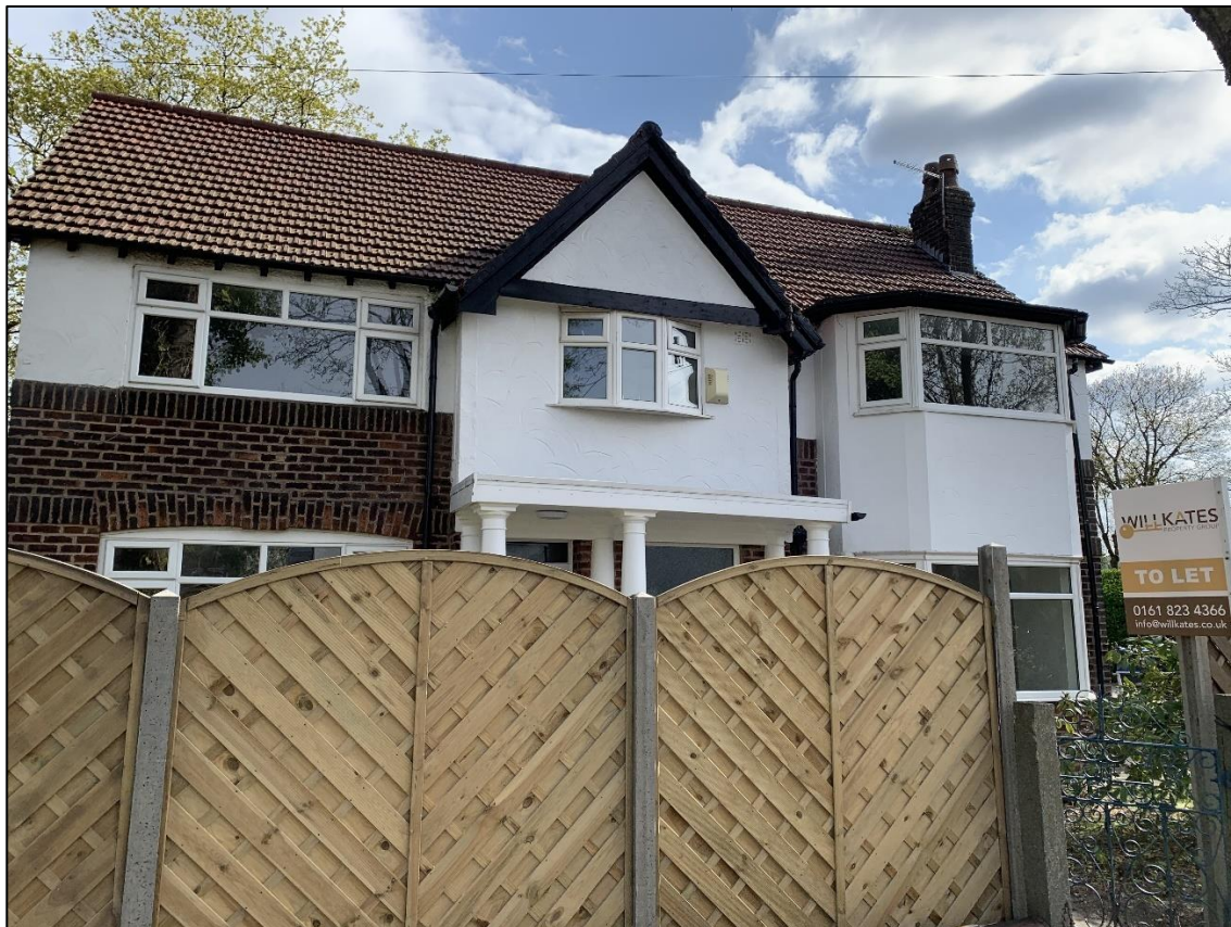
Plate 3 – The south-western elevation of the building
