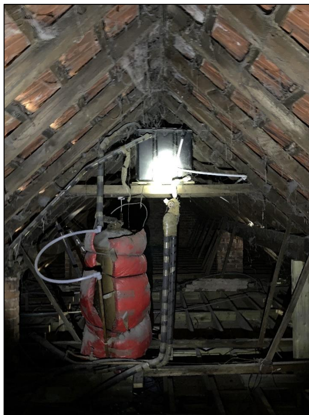
Plate 11 – A further angle of the loft space, showing the water tank and boiler
