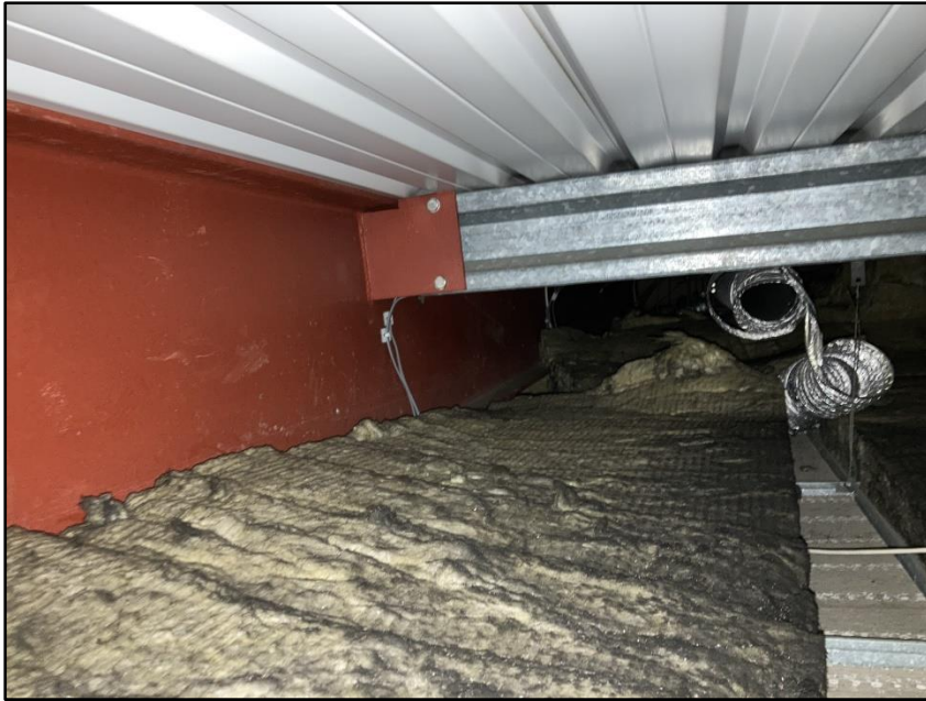
Photograph 38 showing the small roof void space in Building 6
