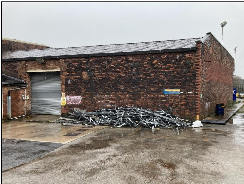
Photograph 39 showing the exterior of Building 7
