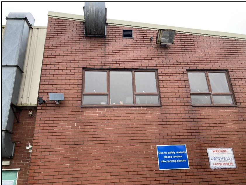
Photograph 31 showing a section of Building 6's exterior
