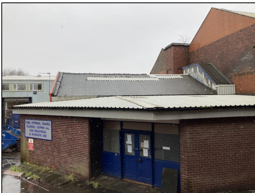
Photograph 17 showing the sloped and pitched roofs of Building 3
