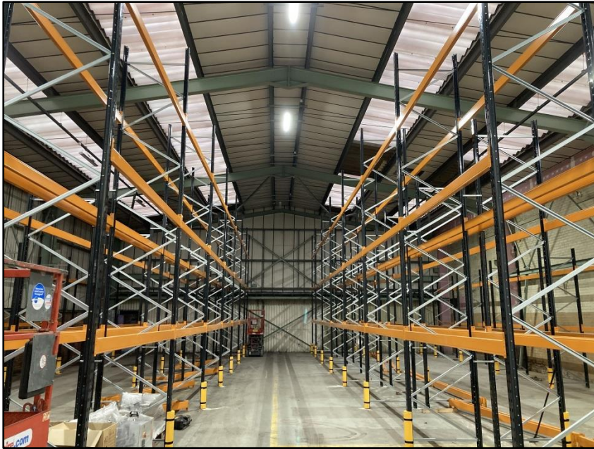
Photograph 11 showing the warehouse section of Building 1
