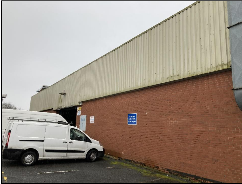
Photograph 32 showing a section of Building 6's exterior
