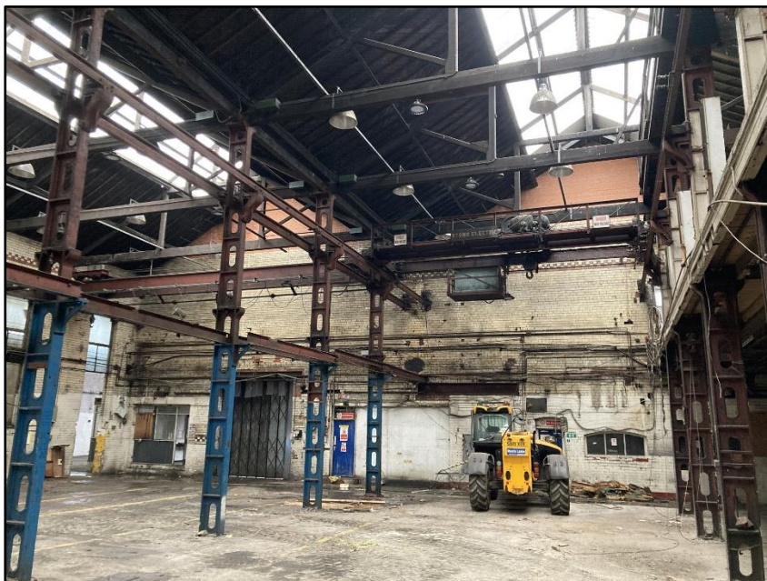
Photograph 22 showing the interior of Building 4
