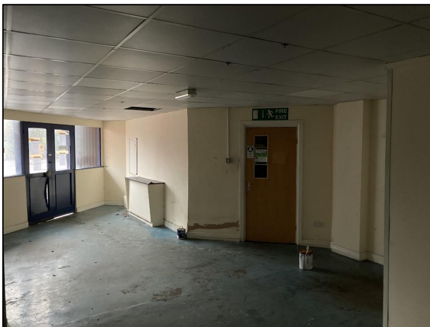
Photograph 19 showing the interior of Building 3
