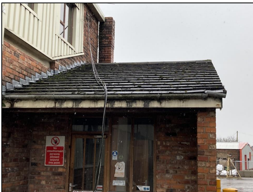
Photograph 34 showing the roof
