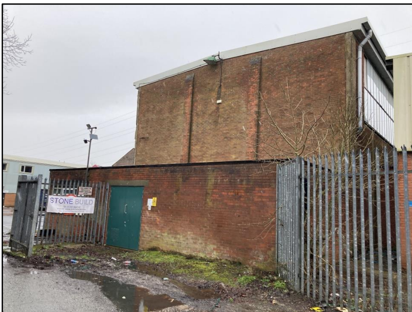
Photograph 27 showing the single-storey part of Building 5
