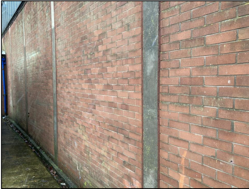
Photograph 26 showing the exterior masonry of Building 5
