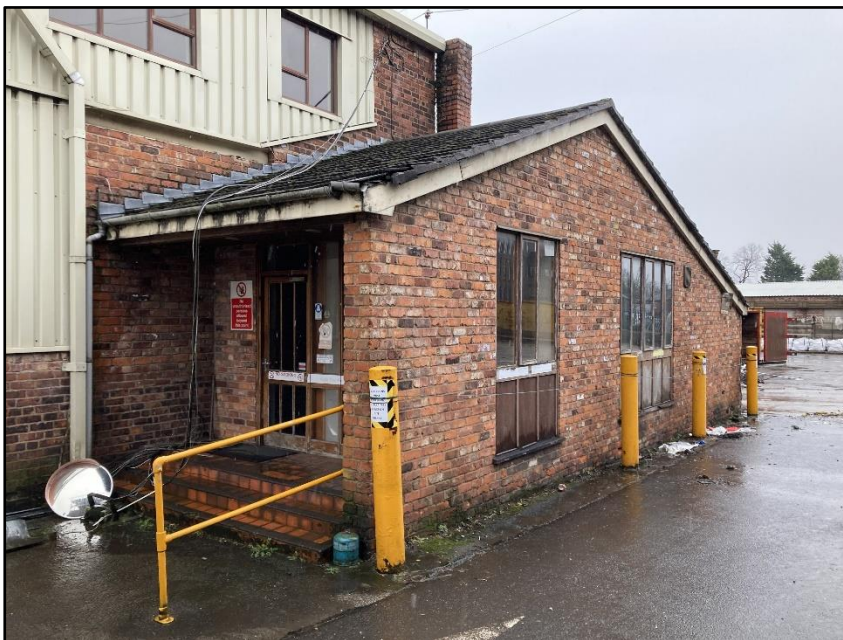
Photograph 33 showing the single storey entrance on Building 6
