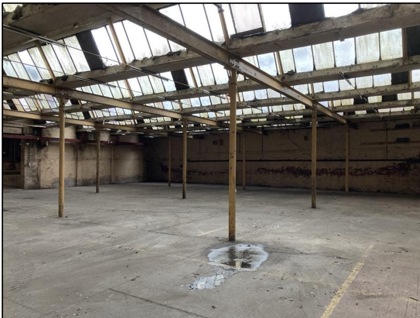
Photograph 41 showing the interior of Building 7
