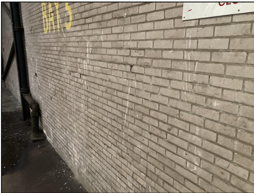
Photograph 37 showing the interior of Building 6
