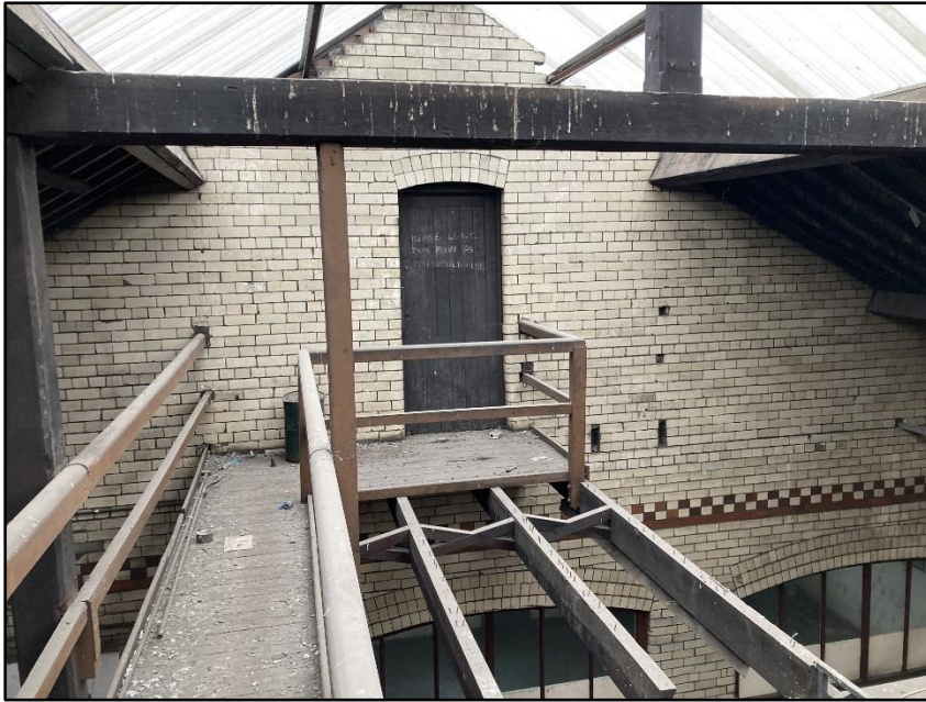
Photograph 24 showing the small room above the office space in Building 4
