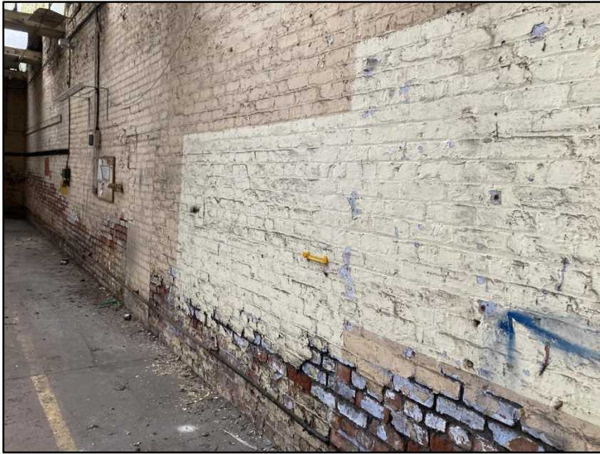
Photograph 42 showing the interior of Building 7
