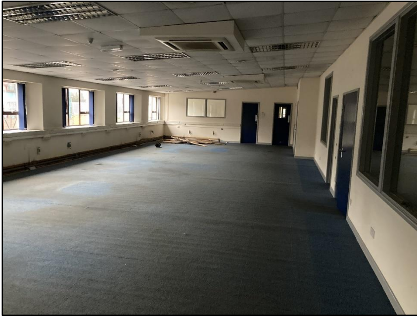
Photograph 36 showing the interior of Building 6
