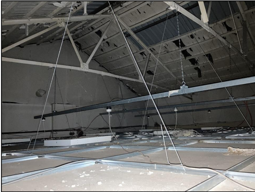
Photograph 20 showing the roof void in Building 3
