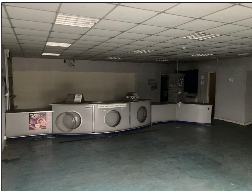
Photograph 18 showing the interior of Building 3
