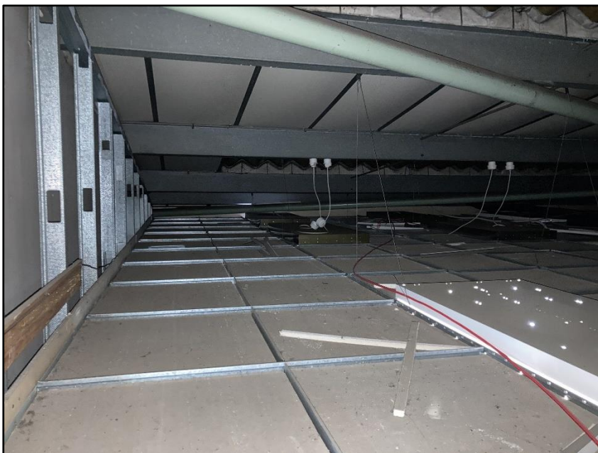
Photograph 10 showing the void space between the suspended ceiling and the underside of the roof in Building 1
