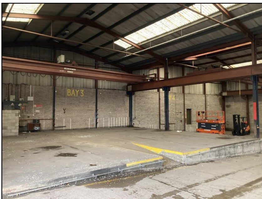
Photograph 35 showing in the interior of Building 6
