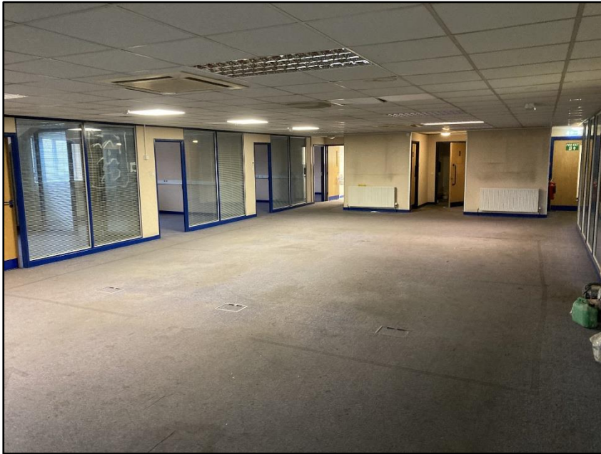
Photograph 9 showing the office spaces in Building 1
