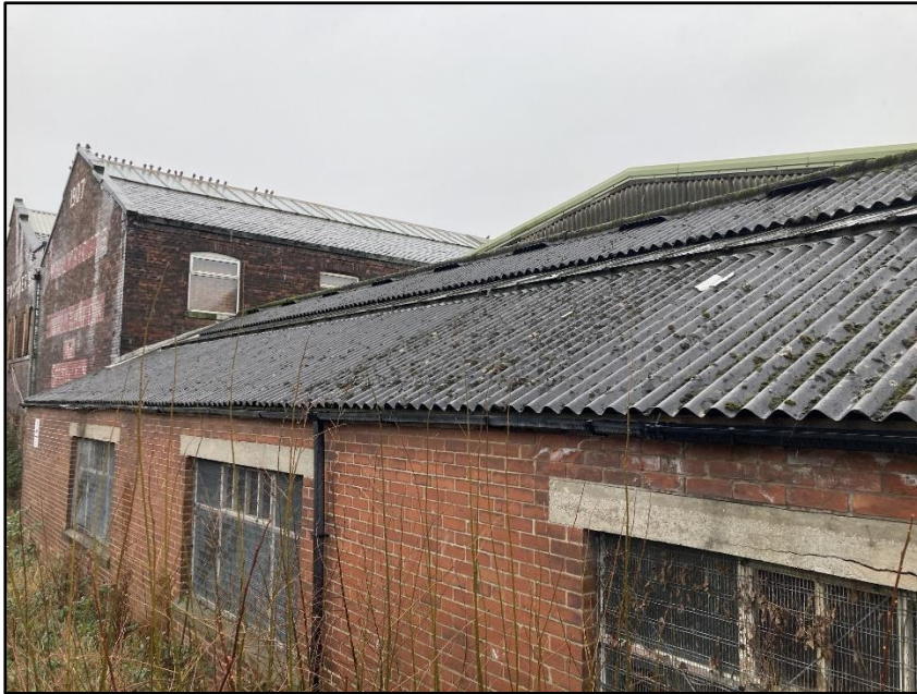
Photograph 14 showing the roof of Building 2
