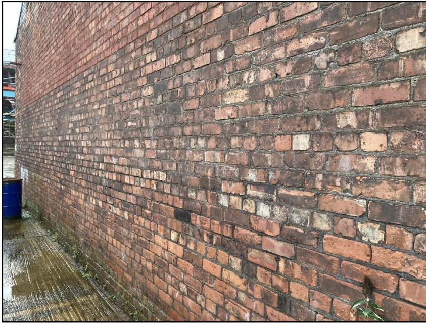
Photograph 40 showing the exterior of Building 7
