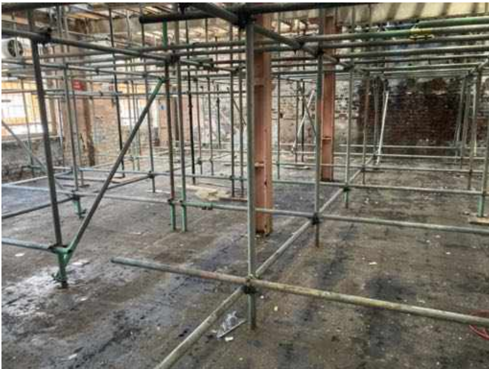
Photograph 12 Description: Ground floor level within on-Site building Date: 10/01/2024 Location: Eastern part of the building
