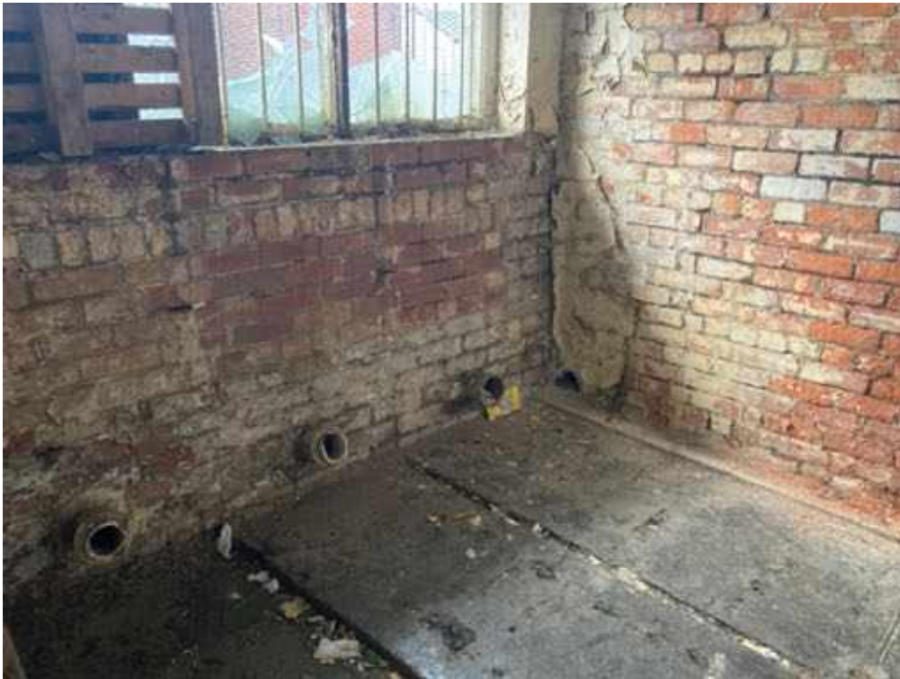
Photograph 11 Description: Former toilet block within on-Site building Date: 10/01/2024 Location: Southern edge of the building
