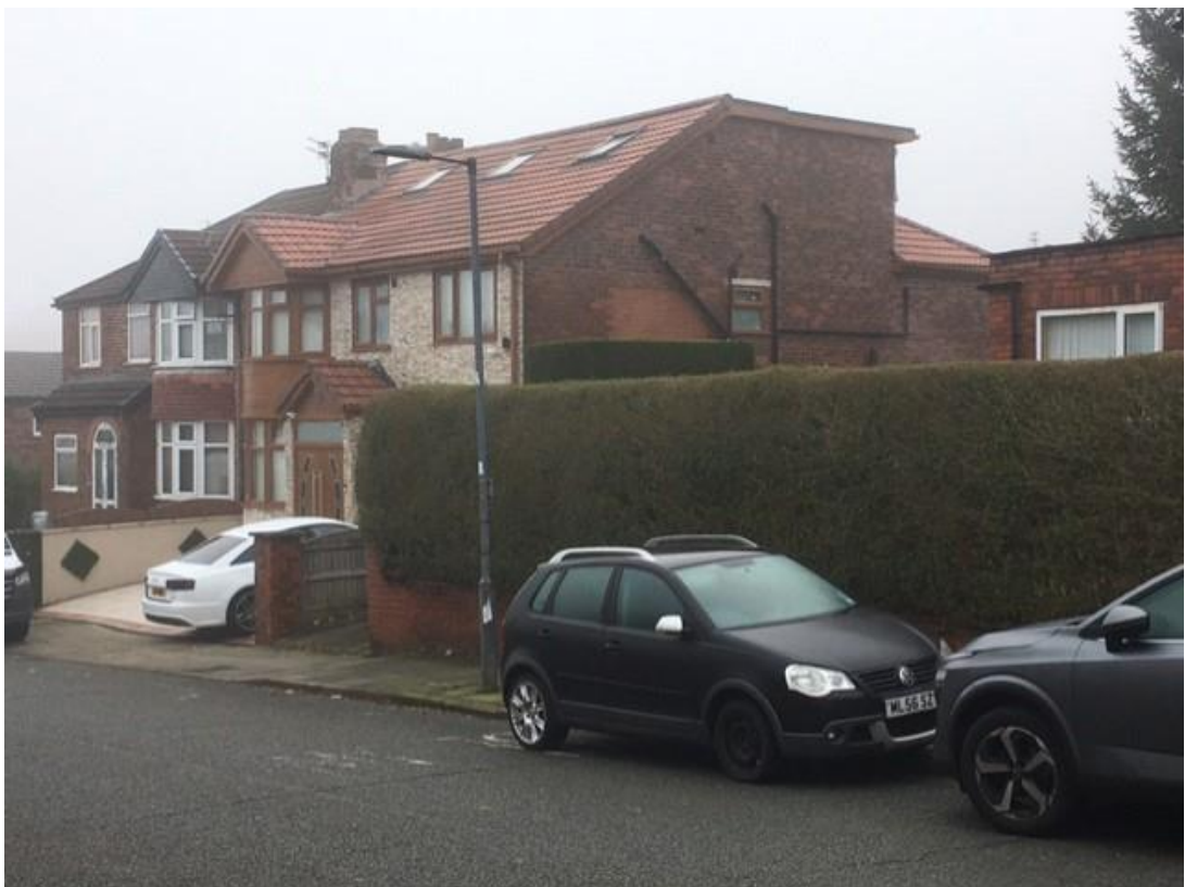
Image 5 – Photo of front and side elevation of property from Windsor Road
