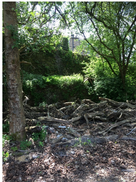
Figure 5: View southwest of debris and retaining walls.
