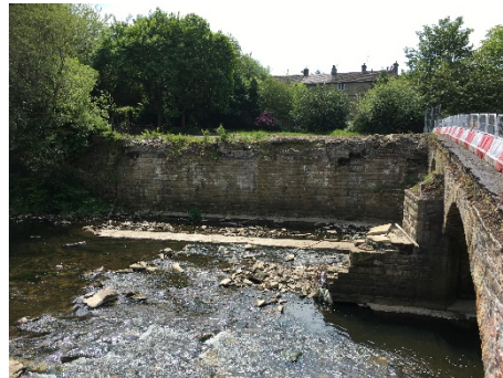
Figure 3: View south of the site and retaining wall.
