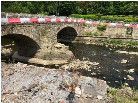
Figure 2: View north of location of the historic Waterside public house and Kay Bridge.
