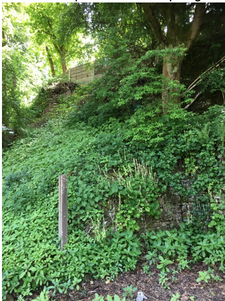
Figure 4: View southeast of slope and retaining wall.
