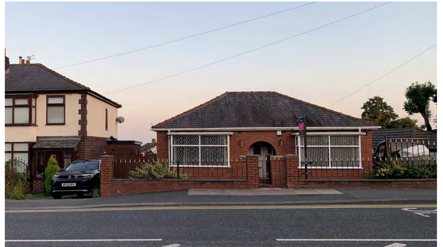
Above: Existing House - Front
