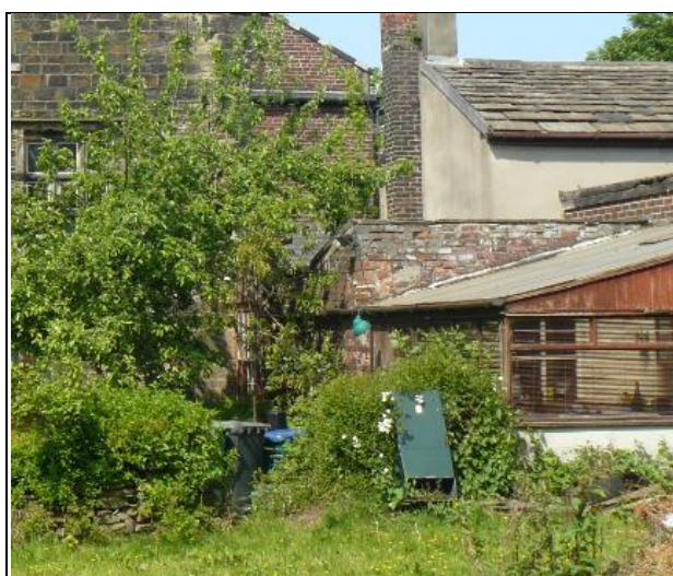
Later Brick Extension with Conservatory Extension in Front
