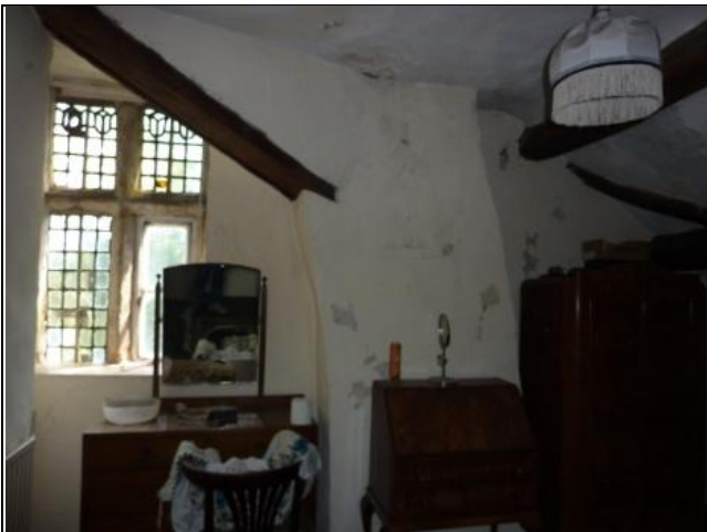
View into Southeast Bedroom
