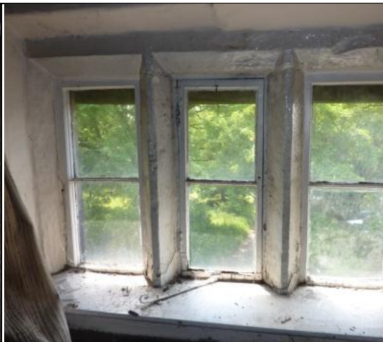
Window in Southwest Bedroom
