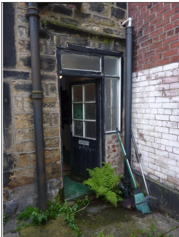
Door and Altered Opening in North Elevation
