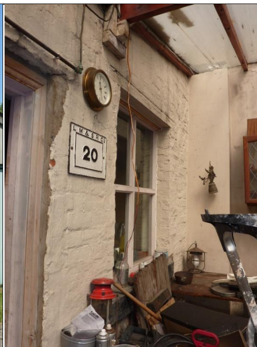
Later Brick Extension Viewed from Conservatory
