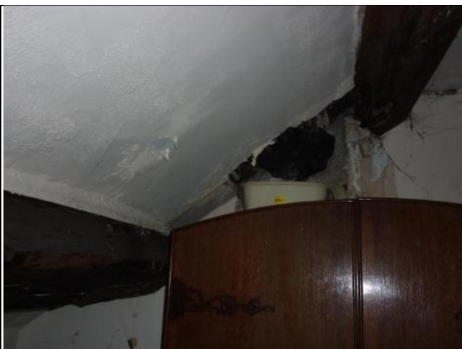
Ceiling in Southwest Bedroom
