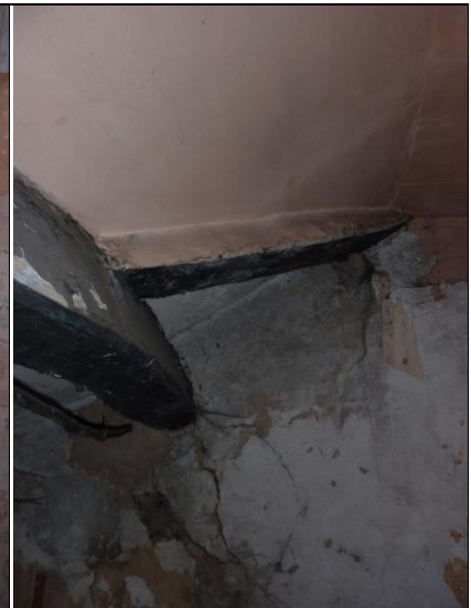
Roof Purlin and Cross Brace
