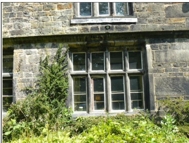
Window on Ground Floor of South Elevation
