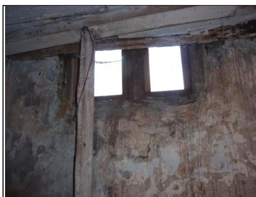
Bottom Window of Stair Window in Basement
