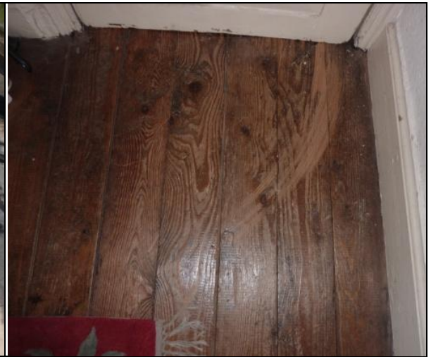
Floor in Southwest Bedroom
