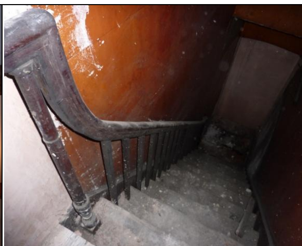
Redundant Staircase Down to Ground Floor
