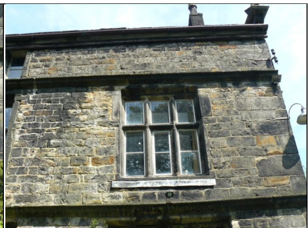
Window on First Floor of South Elevation
