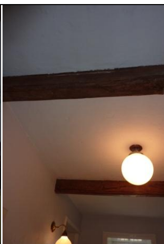
Ceiling in Bathroom
