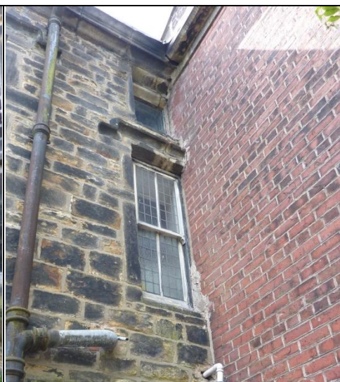
First and Second Floor Windows
