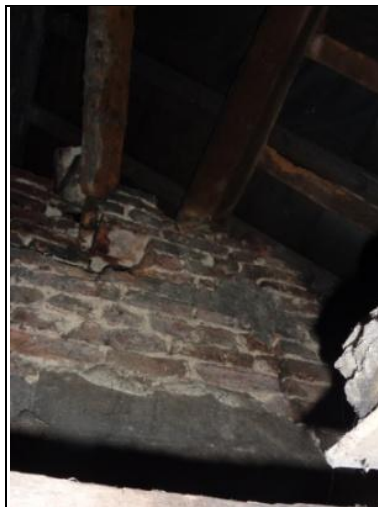
View of Roof through Access Hatch
