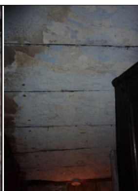
Floorboards and Timber Beams of Basement Ceiling
