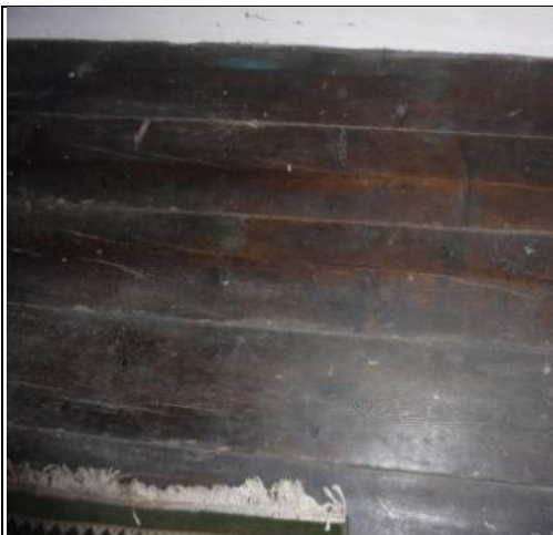
Floor in Southeast Bedroom
