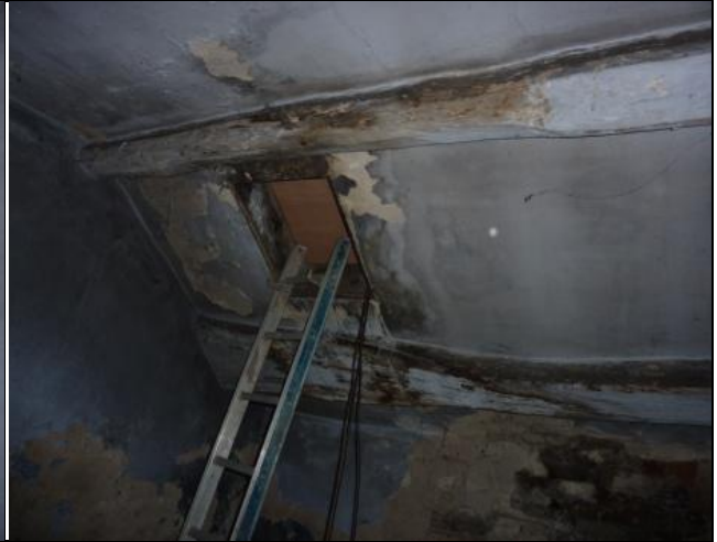
Ceiling in Attic
