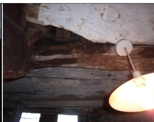
Floorboards and Timber Beams of Basement Ceiling
