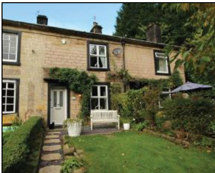
Figure 2: Front elevation 5 East View prior to explosion (2019)
