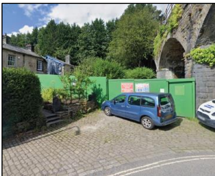
Figure 3: View of cleared and boarded site
