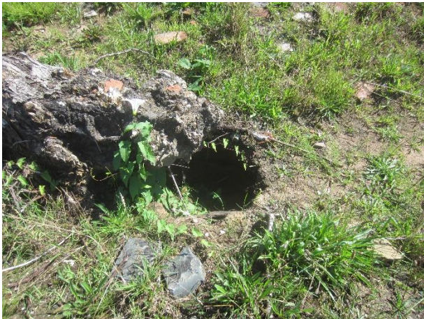
Photo 5: Hole at collapse tree root void near to former fox den
