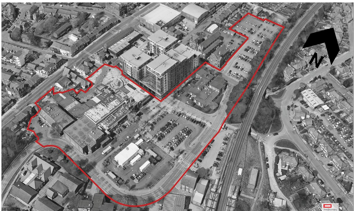
Image 1.1: Aerial View of the Site
