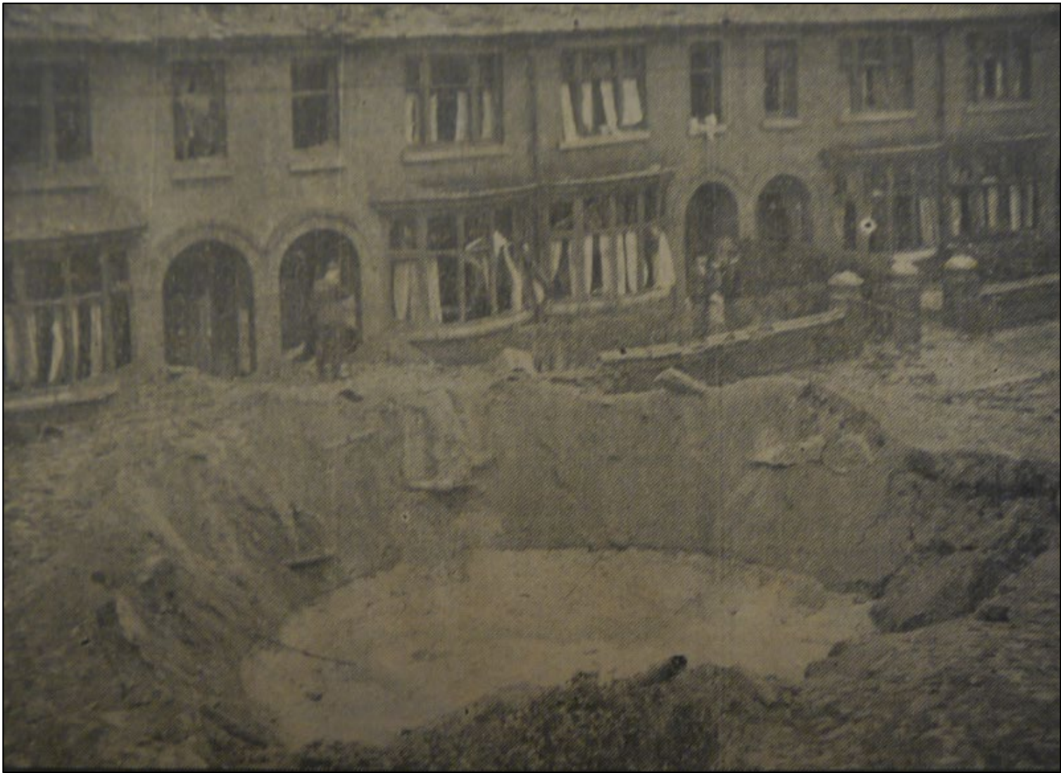
Photograph No.1. During a raid on October 1st, 1940, a heavy bomb caused a deep crater in the centre of the road at the junction of Circular Road and Bland Road, temporarily dislocating the water and sewer services; a heavy stone manhole was hurled some distance away. Although many windows and several doors were blown out the walls of the houses remained intact, except for a few cracks, and damage to the roofs from falling debris. The cheerfulness of the people living in the houses, in spite of any shock they had sustained, was very noticeable. There were no casualties.
